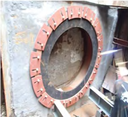
Water-tight Tunnel Entrance Ring with rubber seal
