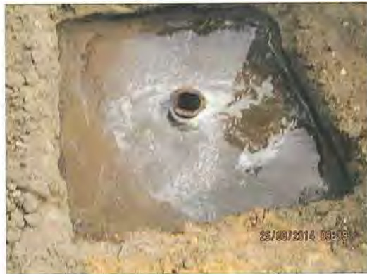
Permeability field test
