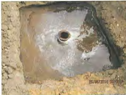
Permeability field test
