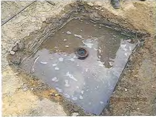
Permeability field test
