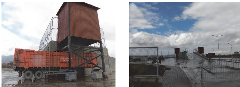
Photo 4-2: Waste transfer station (Türkelit)
