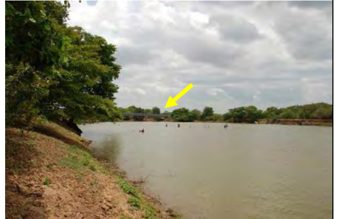
Plate 56. Mahaweli river between AP 7 and AP 8, the bridge on the ring road is in the background of the photo
