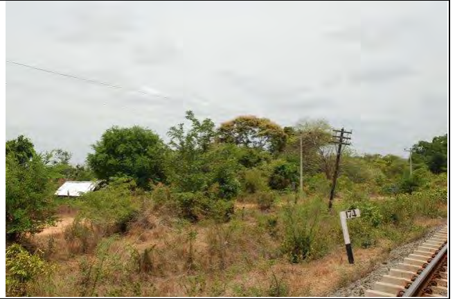
Plate 112. The transmission line crosses the railway line between AP 17 and TT2
