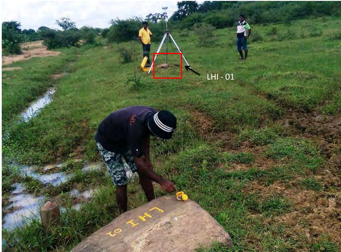
Figure A4 - 3: Establishment of Control Point “LHI01”
