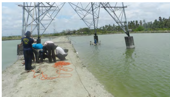
Figure 4.3-16 Long Chimney Foundation (Existing CEB T/L)
