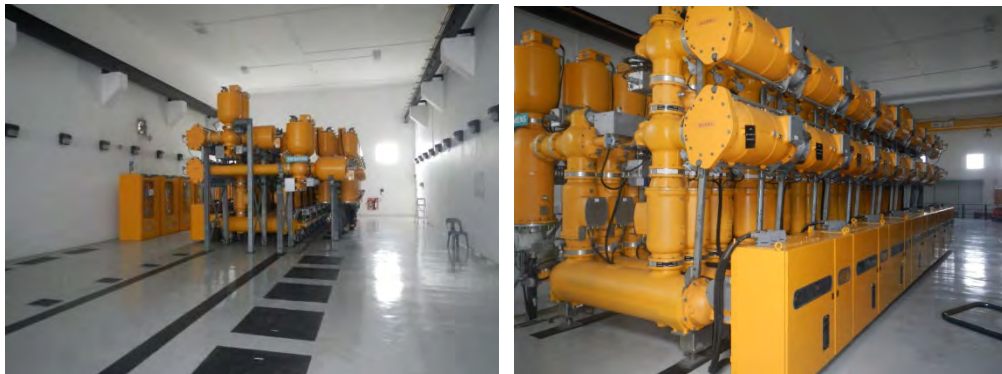
Figure 5.2-2 Indoor Type GIS in the Kerawarapitiya S/S
