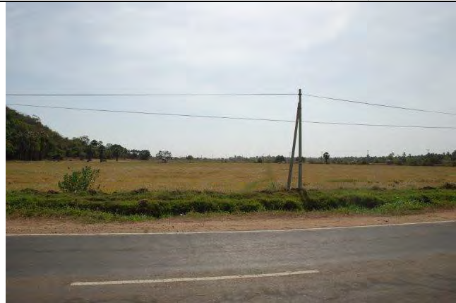
Plate 41. Transmission line crosses Trincomalee-Muthur- Batticaloa road (coordinates: 08.412717, 81.264962)
