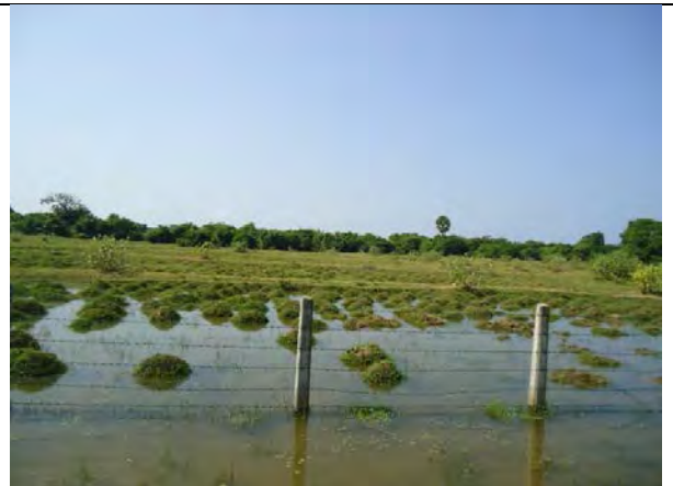
Water Logged area in the Project site
