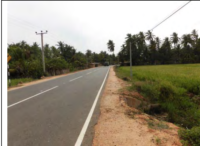
Plate 91. The transmission line crosses the Tambalagamuwa- Kinniya road
