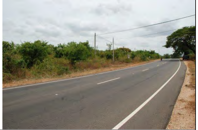
Plate 122. The GSS land bordering the Habarana-Trinco A6 road (300 m along the road x 225 m towards the teak plantation)
