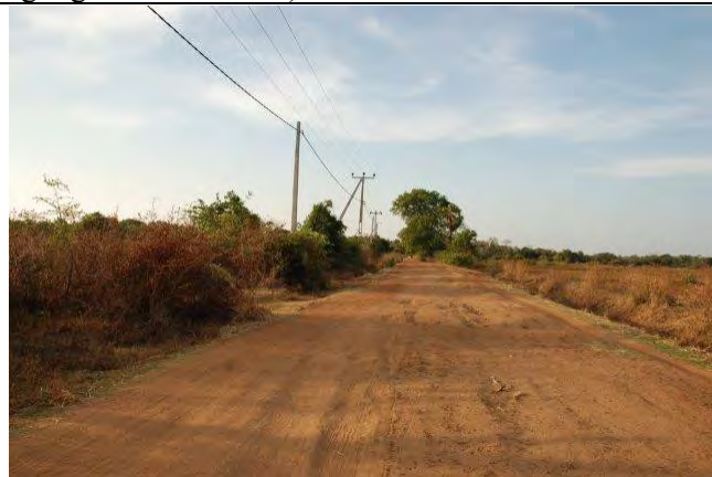
Plate 29. The ring road start from Soorungal (Mullipotana- Surangal road) and ending at Illakanthai. The angle points 4 to 12 are located either side of the road.
