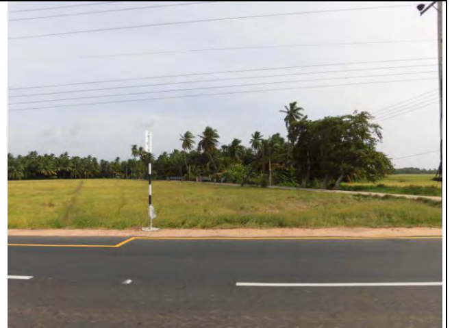
Plate 92. The transmission line crosses the Tambalagamuwa- Kinniya road
