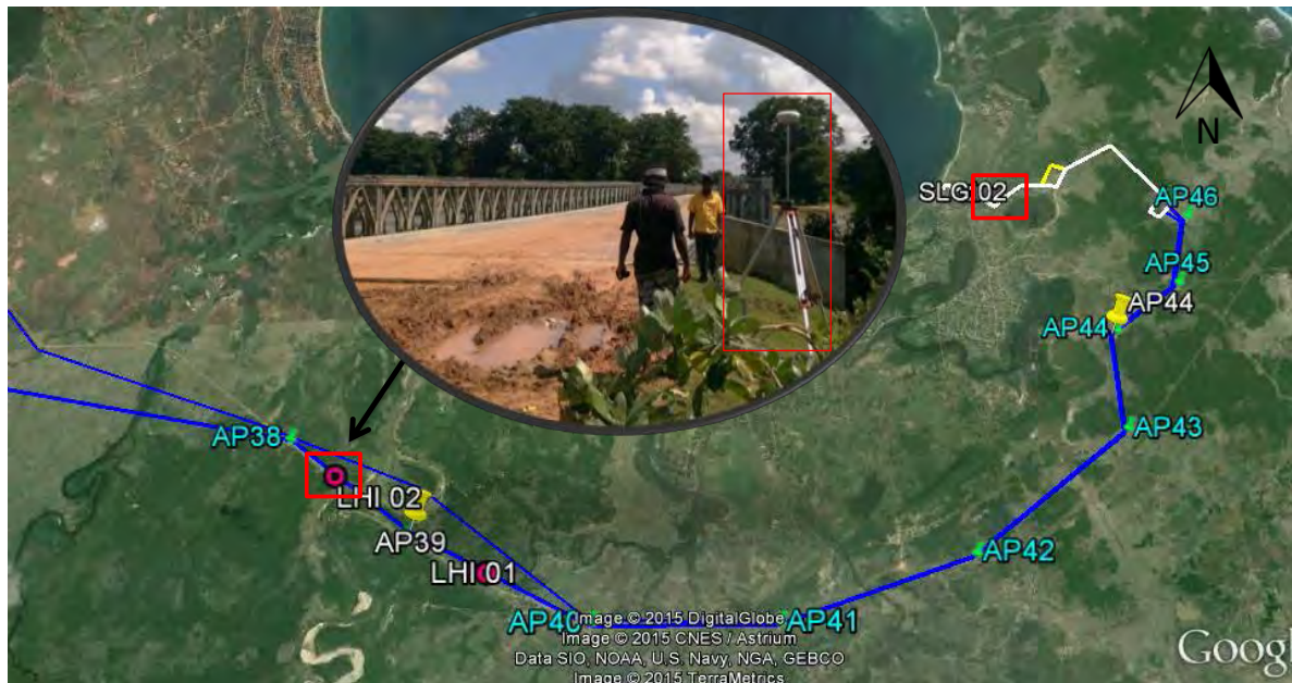
Figure A4 - 4: Control Point “LHI02”
