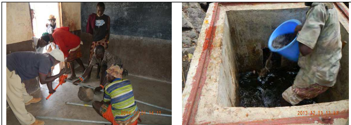
Figure AD3.5.1 Technical Transfer on Maintenance of Pipeline: (left :community members being trained on pipeline maintenance, right: a community member cleans the catchment at the springs)
