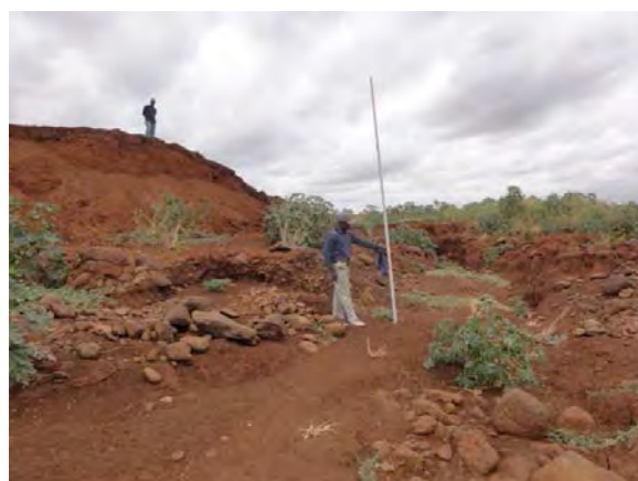
Figure AD2.4.2 Damages by Scouring Dololo Dokatu Water Pan
