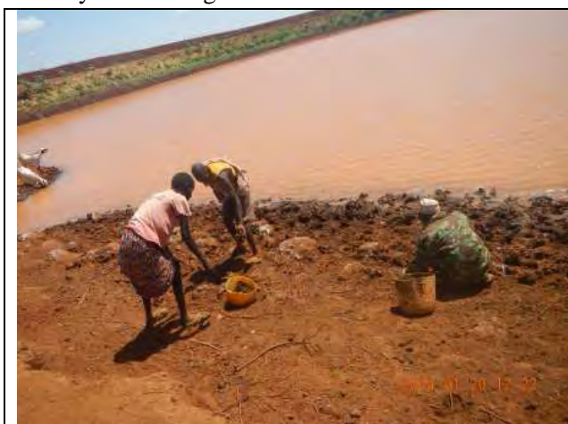
Figure AD2.7.2 Herders Desilt and Collect Dung from the Watering Point at Dololo Water Pan
