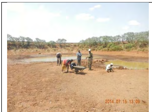
Figure AD2.7.3 Desilting Work by the Community at Dololo Water Pan
