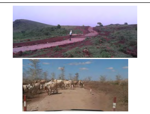
Rural Road Improvement - upper: Hurri Hills, lower: Ngurnit (Marsabit)
