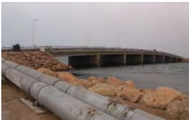
Figure TR 1-10-7 Opening by bridge on the Chaussée romaine
