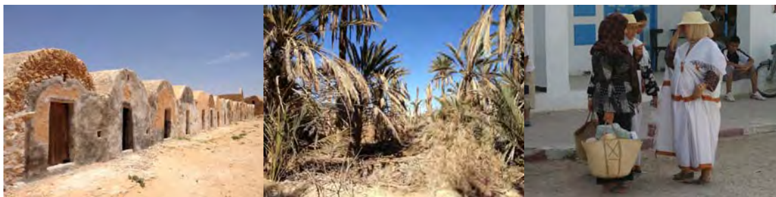
Ksour restored by inappropriate materials (Tataouine)
