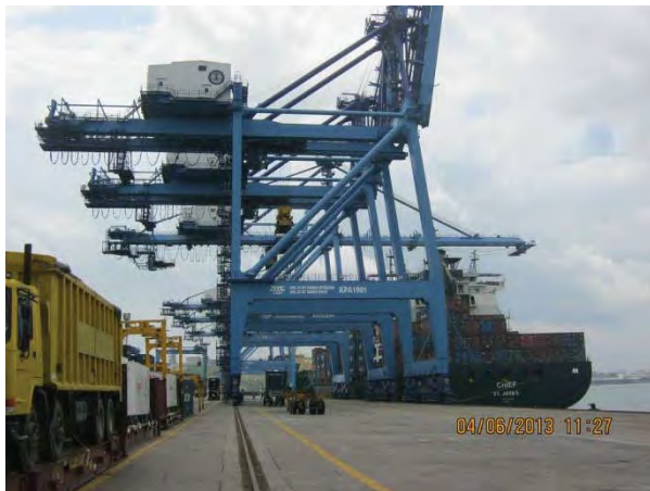
Berth 19 and Ship-to-shore Gantry Cranes
