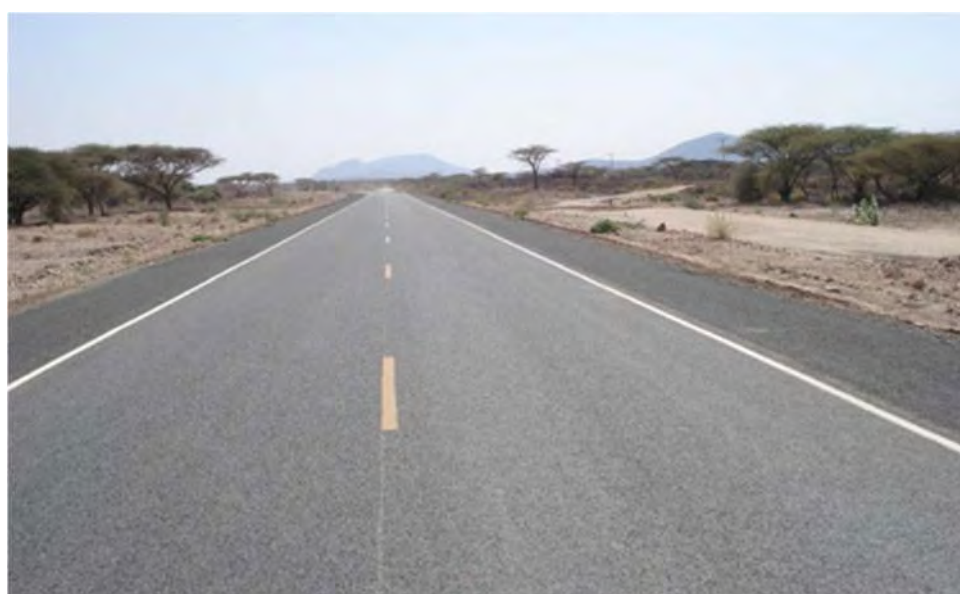
Figure 3.4.12 LAPSSET Road (Isiolo-Moyale section)
