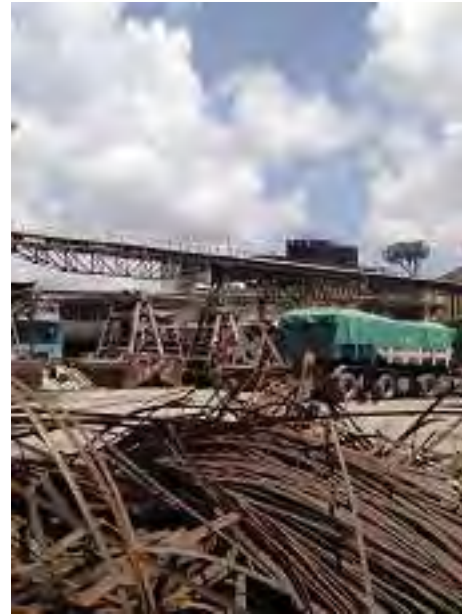
Belt Conveyor for Soda Ash
