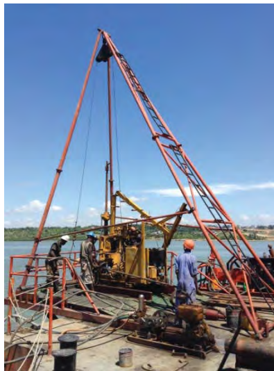
Drilling Rig (Offshore)
