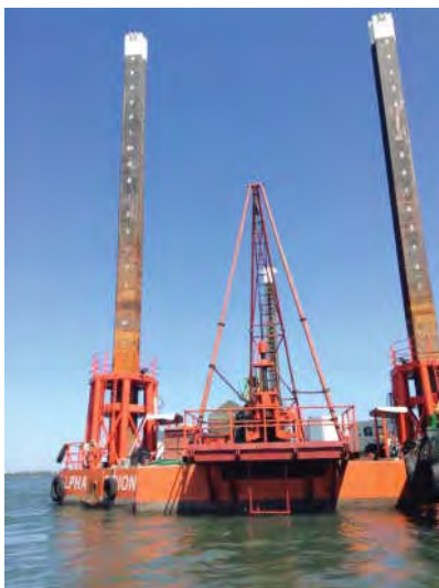
Jack Up Barge (Pontoon)
