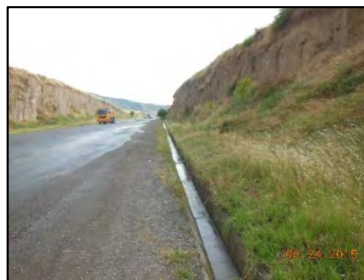
(b) Concrete Ditch
