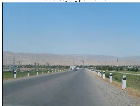
Concrete Post Only at Embankment Section (No cables)
