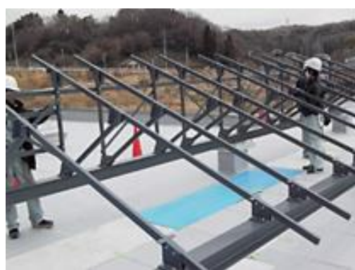
Figure 3-13 FRP PV frame (Cosmo System website)
