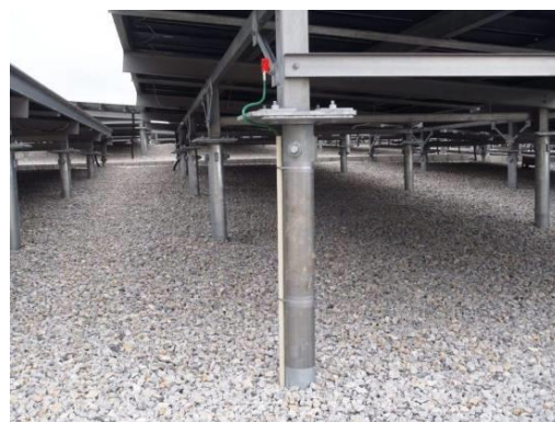
Figure 3-11 Spiral steel pipe pile (Abe Mega Solar Demonstration Research Facility PV foundation)
