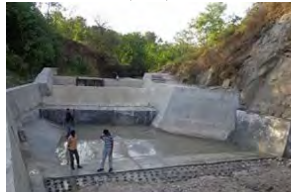
Intake Structure and Downstream Apron (Phase1)
