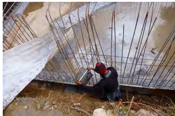
Curing of water tank (Phase1)
