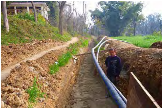
Laying of HDPE pipe (Phase1)
