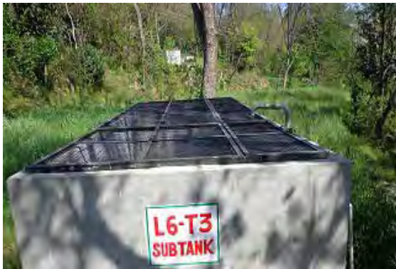
Irrigation facilities (Phase1)
