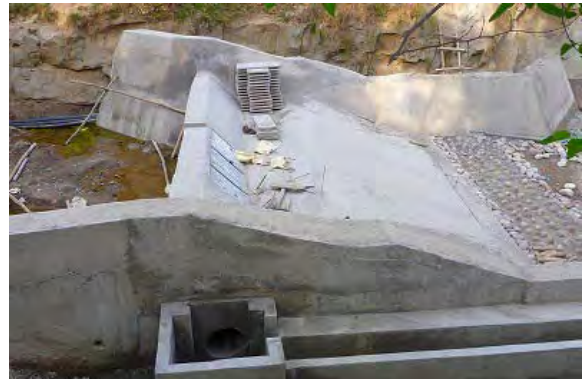
Under construction of intake (Phase1)
