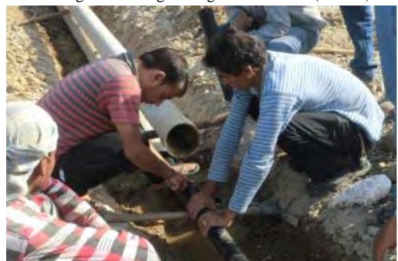
Field support to GMKVA Repair of pipeline leakage (Phase3)
