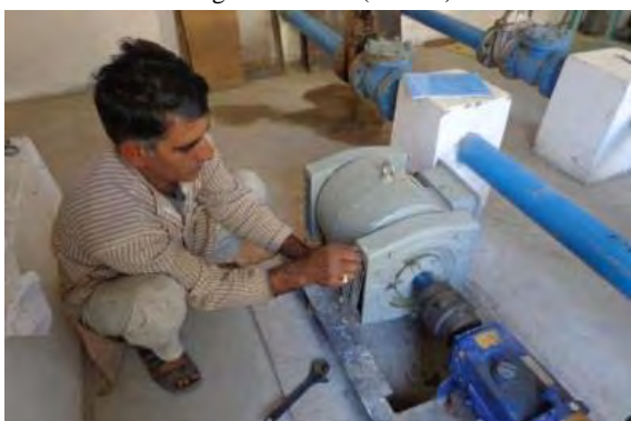
Field support to GMKVA Maintenance of pumping facilities (Phase3)
