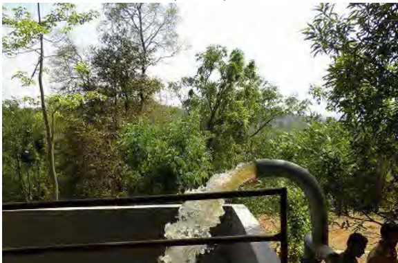
Test run (Phase1)
