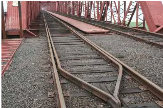
Although the Bangabandhu Bridge is not equipped with derailment prevention guards, this bridge is equipped with derailment prevention guards.
