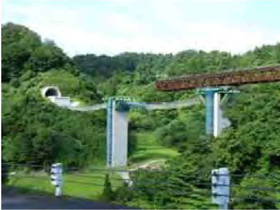
[Fig. 4.1.4] Truss girder launching erection method
