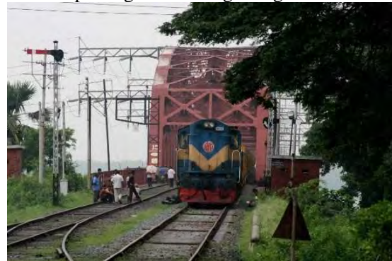
This bridge was constructed as double track bridge. But connecting approach tracks are only single. As wind speed of this area is large, the double track structure was adopted to increase wind load resistance.
