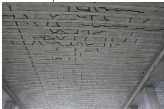
RC Slab Bridge. Many cracks are developed on the bottom slab.
