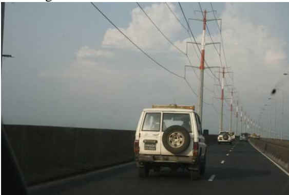
End section of four (4) lane road is occupied by train track and lanes became narrower. Beyond left concrete barrier, a rail track exists.
