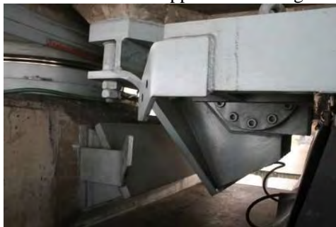
25. Lateral movement stopper and bearing
