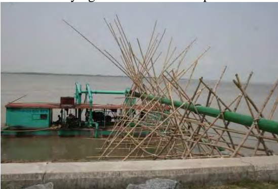
Sand is pumped up from ship to bank.
