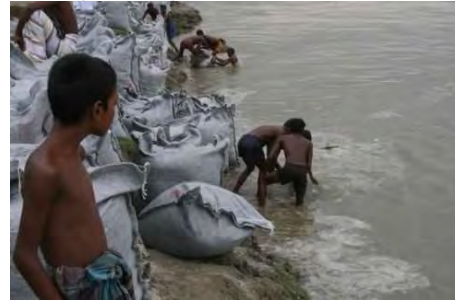
Manual sand bag sinking
