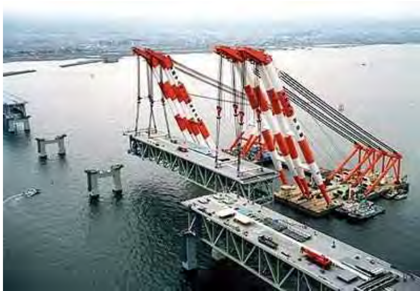
[Fig. 4.1.6] Large block erection method by floating crane, Kansai Airport Access Bridge
