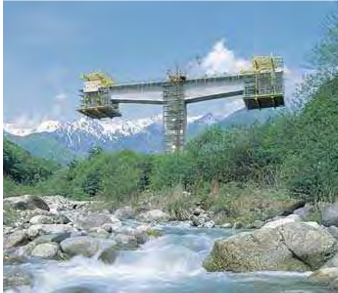
[Fig. 4.1.1] Balanced cantilever method
