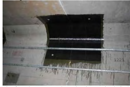
22. Trial repair of cracks
