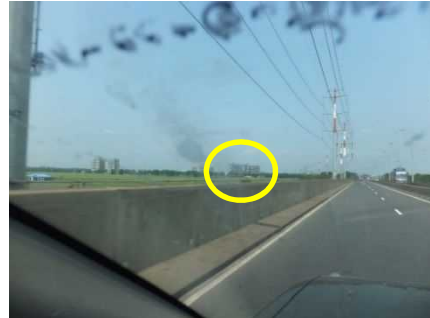
If the new railway bridge alignment is planned slightly more to the north, the train track may interfere with these buildings.
