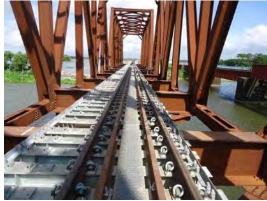
Note: Bridge No.185 (Span 140.3m)
