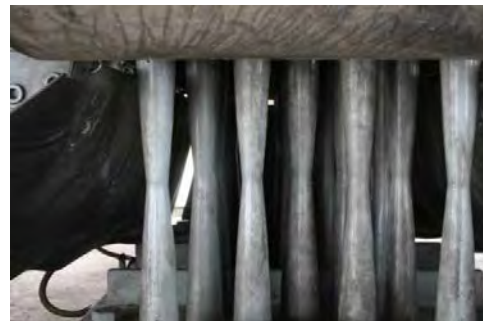
26. Seismic resistance device
