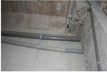
21. Pipes inside of girder
