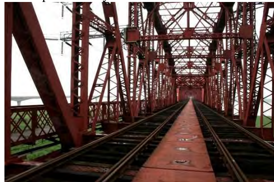
60. Inspection way between tracks
