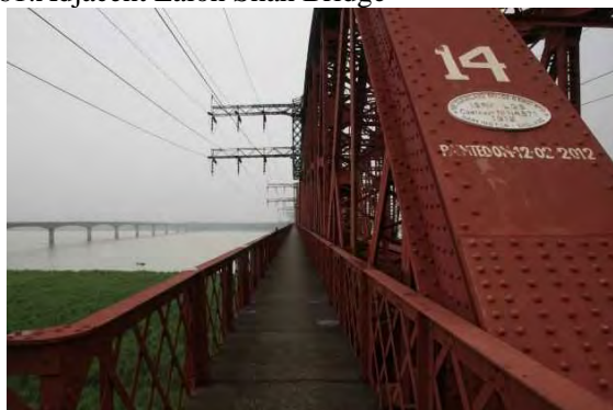
61. Adjacent Lalon Shah Bridge
