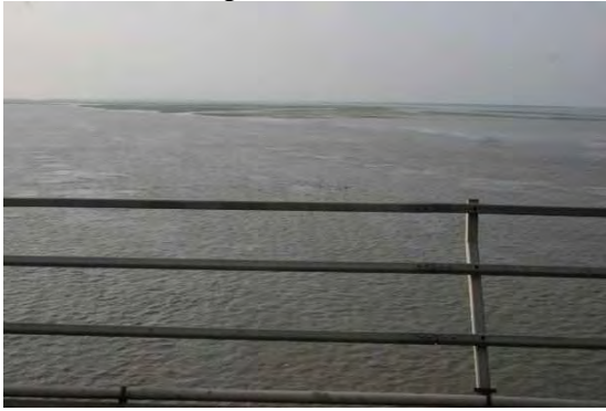
Submerged sand bar upstream of the Bangabandhu Bridge and near planned new railway bridge site
