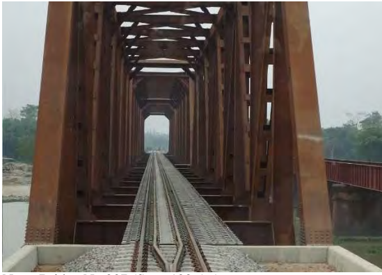
Note: Bridge No.207 (Span 120.5m)
