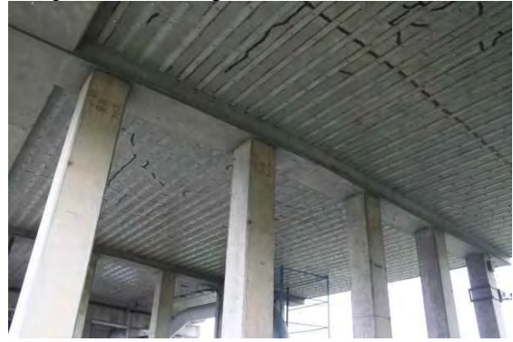
Narrow steel strips in longitudinal direction are attached. Cracks may have appeared in lateral direction.
