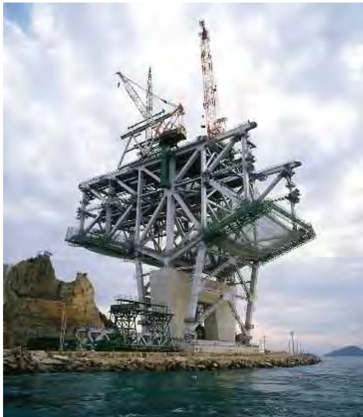
[Fig. 4.1.5] Piece by piece erection of Yoshima Bridge
