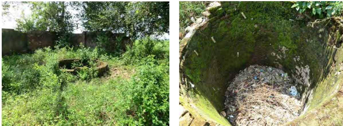
Photo I.2.3 Pit for Risk Waste at BHU
