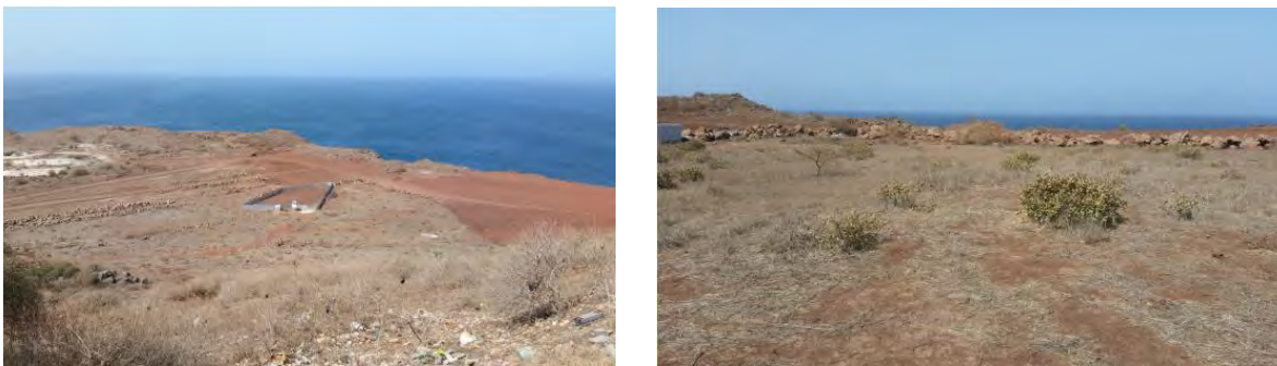
Picture 5.1.1 Current condition of the Construction Area (Left: Panoramic view, Right: Surface soil and some plants)
