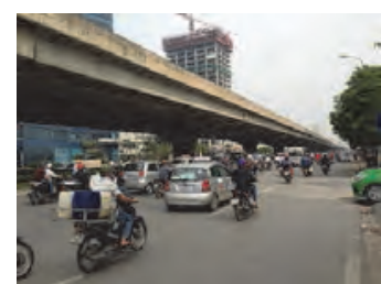
Viaduct on Ring Road 3 at Trung Hoa
