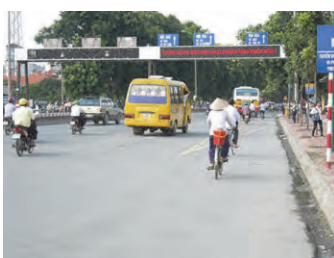
VMS on Ring Road 3 at Mai Dich
