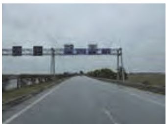
VMS on Ha Noi-Bac Ninh
