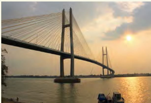
The Tsubasa Bridge from the eastern bank of the Mekong River. The crane used during construction was removed just before the bridge was opened. (Photograph March 2015)
