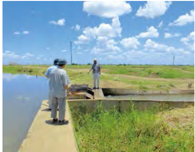
Support for restoring Shokue Irrigation System, destroyed by a flood (Mozambique)
