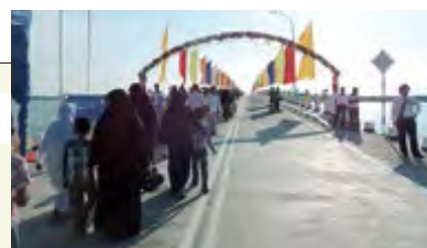
The Manmunai Bridge, completed in April 2014. Many local people attended the opening ceremony.
