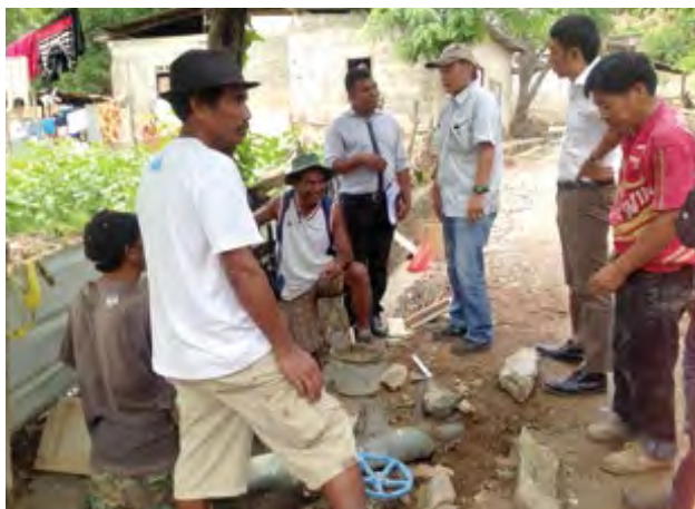
Water supply improvement advisor repairing deteriorated water pipes in Dili (Timor-Leste).
