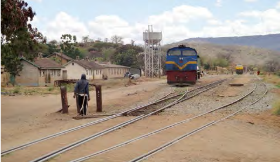
Support for improving the transport capacity of the aging central railway in the Central Corridor in Tanzania. JICA began a preparatory survey for cooperation in July 2014.
