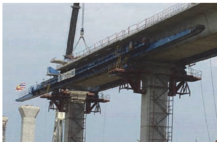
Figure 4.4.9 Example of Construction Method for Girder Erection
