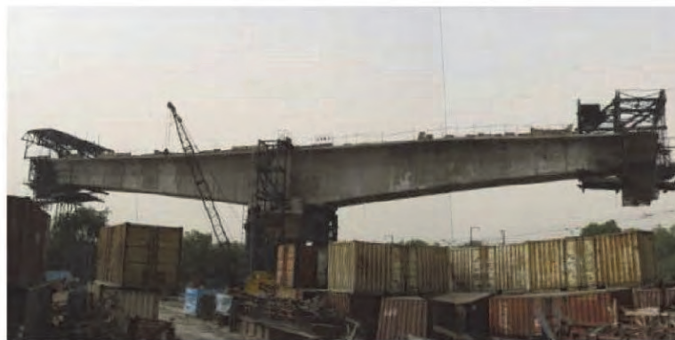
Figure 4.4.12 Long Span Bridge Delhi Metro Phase2, India
