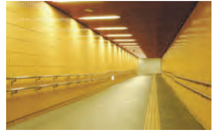
Slope with doubled handrail
