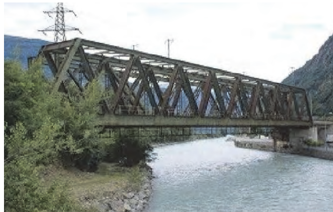
Figure 4.4.14 Photo of Steel Truss Type Girder
