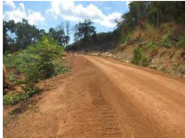
Route of the Penstock
