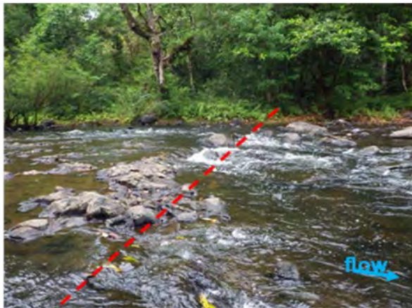
Intake Weir (Right bank :Xe Katam River)
