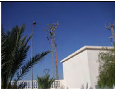
Photo 7 STEG transmission tower
