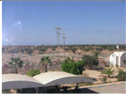
Photo 14 STEG transmission tower
