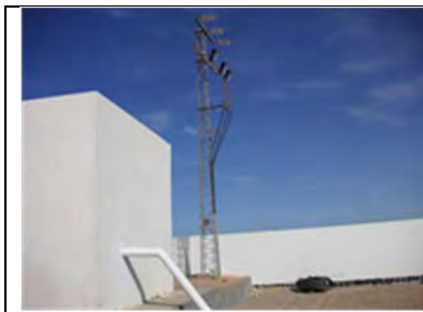
Photo 36 STEG transmission tower
