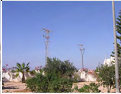
Photo 15 STEG transmission tower
