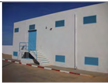
Photo 37 Power receiving room
