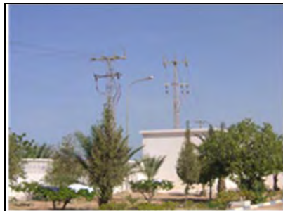
Photo 6 STEG transmission tower
