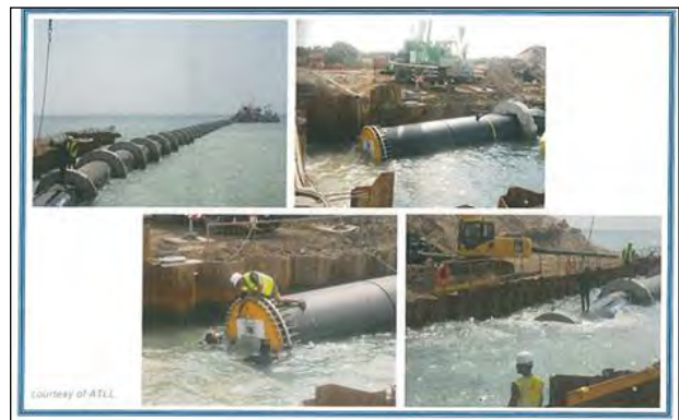
Source: GWI Figure 5.5-4 Steel Pipe Construction
