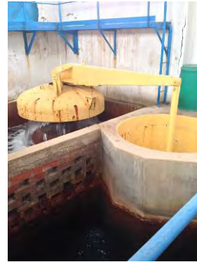
Photo 4 Inside of the mixing basin
