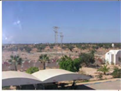
Photo 14 STEG transmission tower
