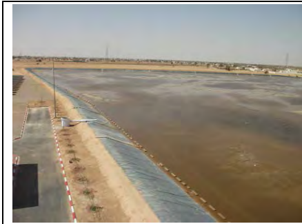
Photo 32 Sun drying bed
