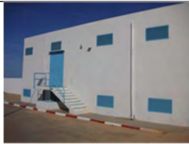
Photo 37 Power receiving room
