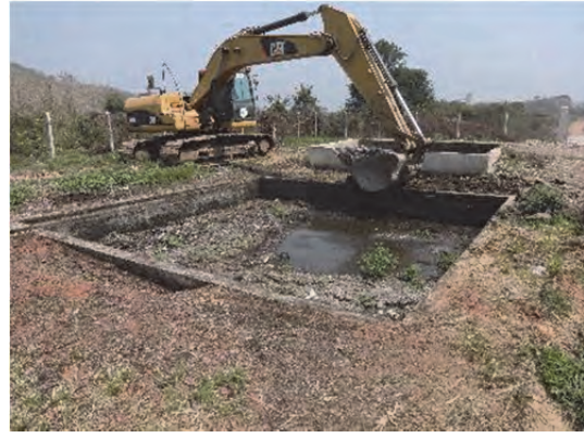
Photo: Removal of sedimentation by excavator (VTE KM32)
