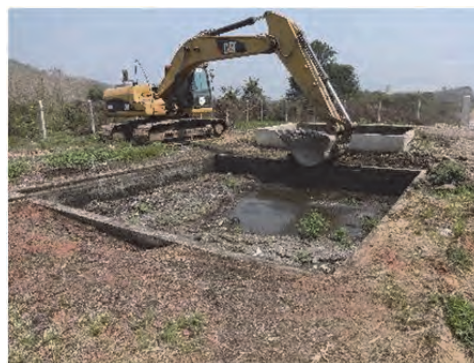
Photo: Removal of sedimentation by excavator (VTE KM32)
