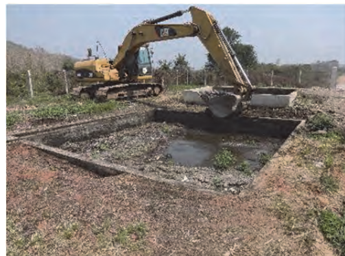
Photo: Removal of sedimentation by excavator
