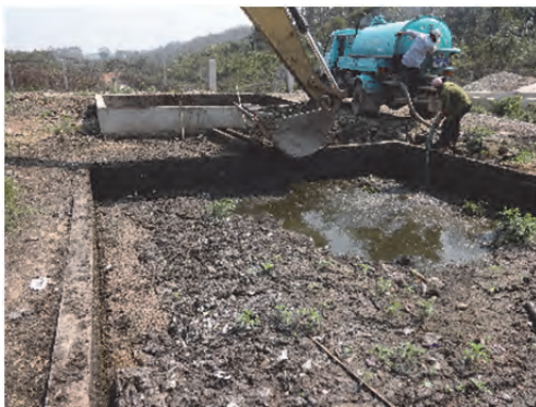
Photo: Removal of sedimentation by excavator
