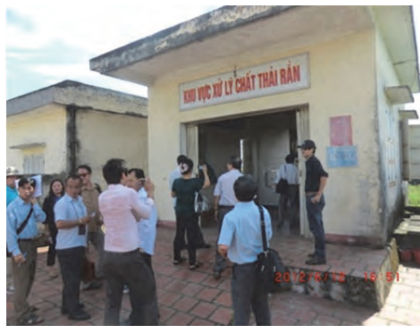
(Thanh Hoa 71 Central Hospital 医療廃棄物焼却施設)
