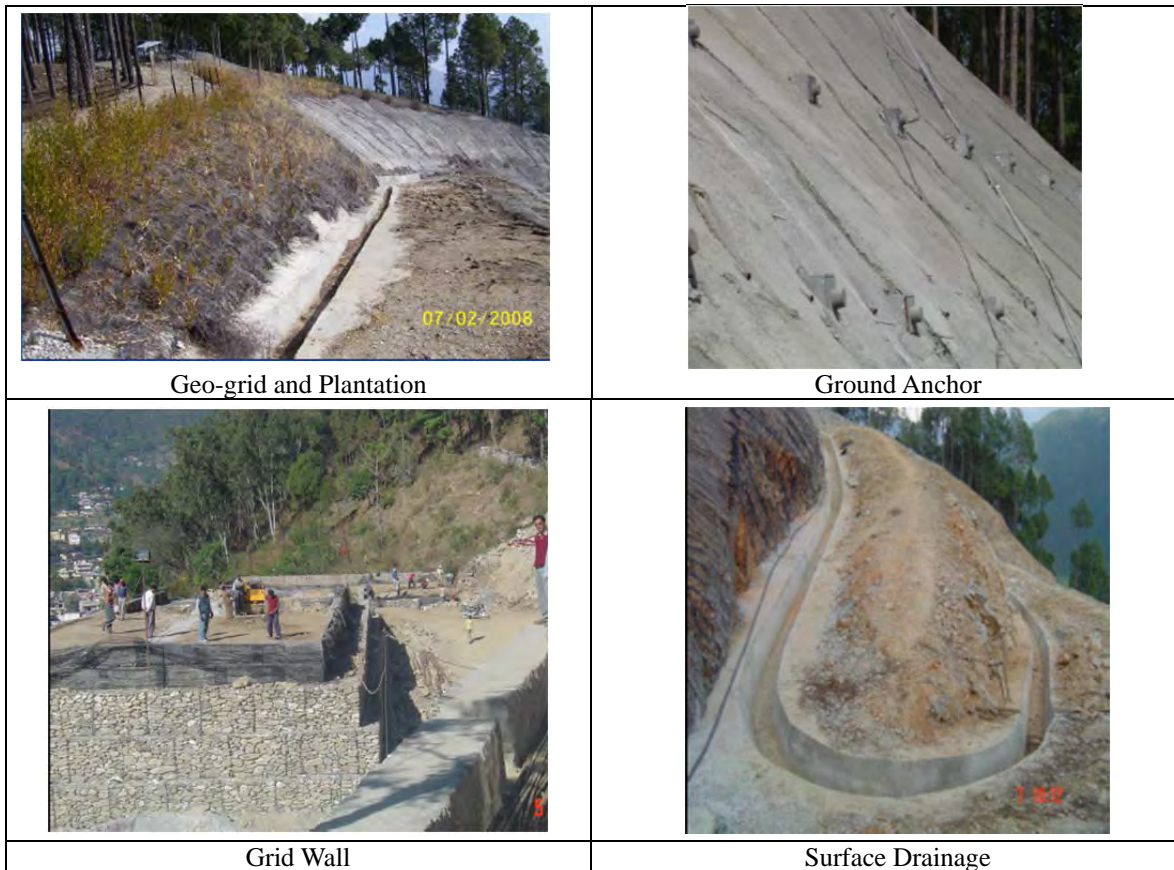
Figure 4.3.10 Examples of Countermeasures for Varnavat Landslide
