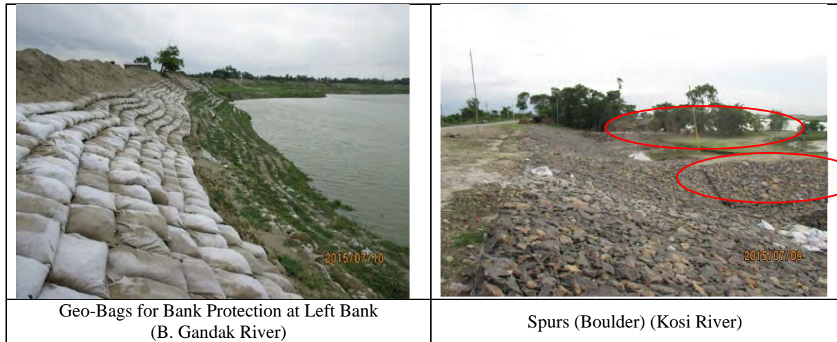
Figure 7.3.17 Adopted Structural Measures for Bank Protection
