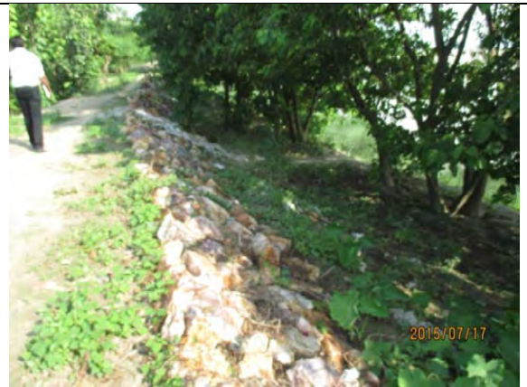
Protection Works by Boulder Pitching Works at Dhamaun (Ganga River)
