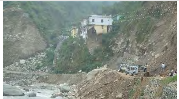
Area eroded by the flood 2013 (at Khagaria, Rudraprayag District)
