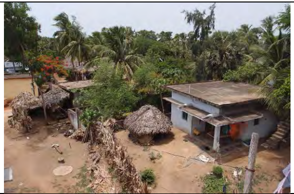
View of Krishna Manda, Krishna District (from the roof top of cyclone shelter)
