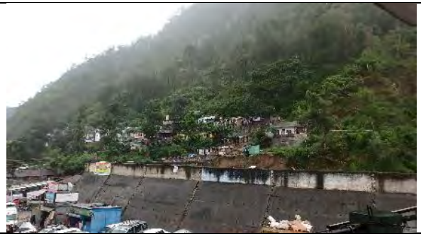
Varnavat Landslide Area (Uttarkashi District)
