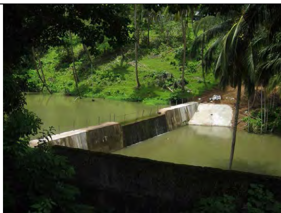
Check Dam near Beadonabad Village
