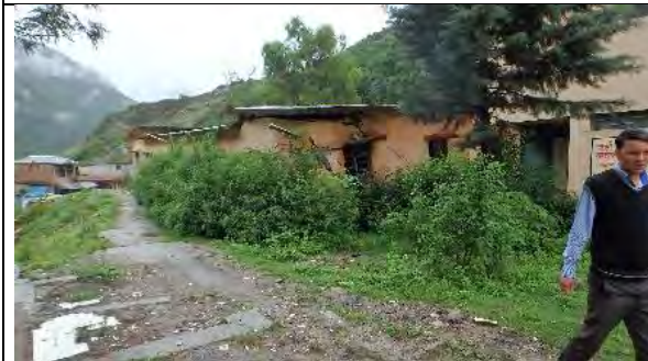
Houses wrecked by Slope Failure along a River (Uttarkashi District)
