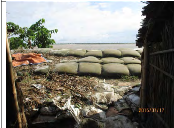
Protection Works by Sand Bags at Dhamaun (Ganga River)
