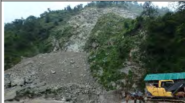
Landslide by the flood 3013 (at Sonprayag, Rudraprayag District)
