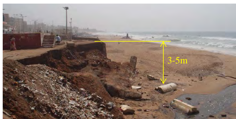
Source: prepared by the Survey Team
