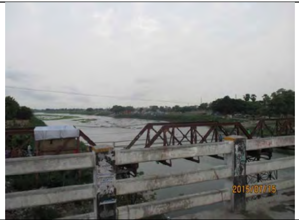
Burhi Gandak River (Samastipur Bridge)
