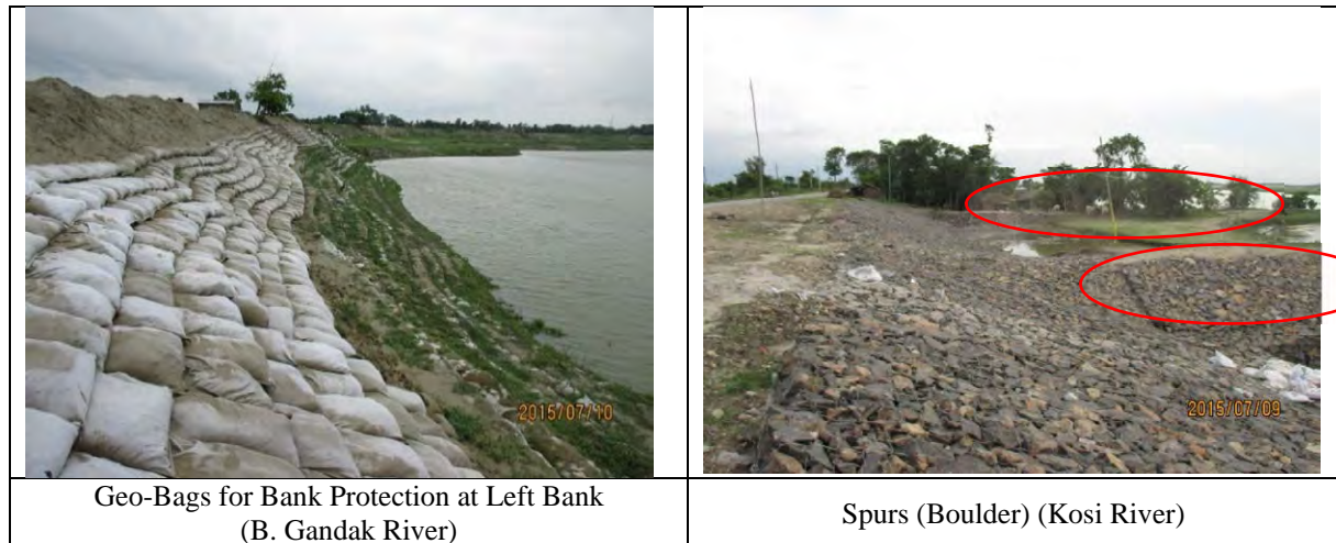
Figure 7.3.17 Adopted Structural Measures for Bank Protection
