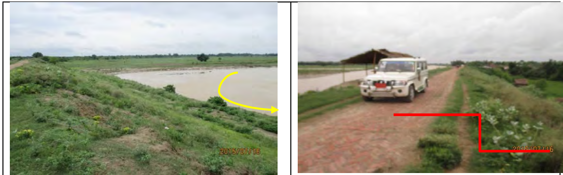
Figure 7.3.16 Meandering of River and Lower Ground than River Water in the Kamla River (Janjharpur District)
