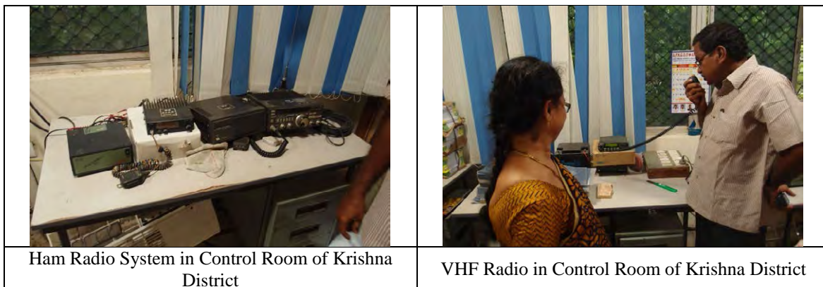
Source: prepared by the Survey Team
