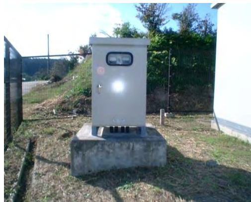
Figure 2.4-23 Installation of Cathodic Protection System (Example)
