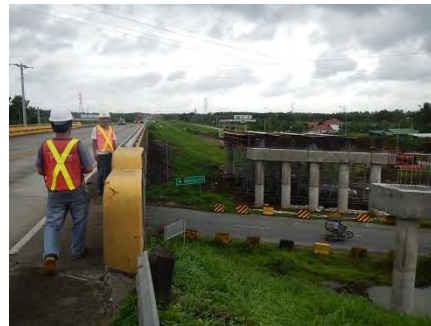
Expansion works (Bridge)
