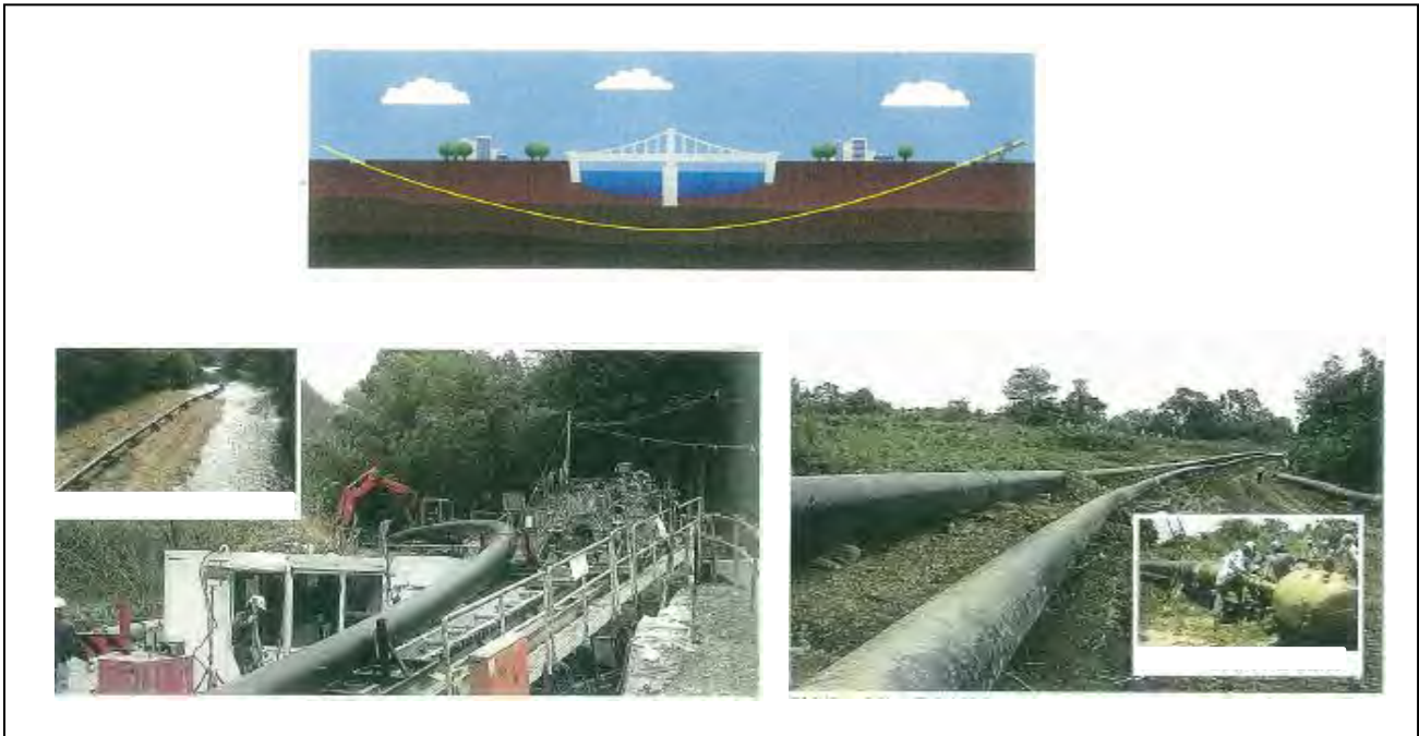
Figure 2.4-51 HDD Method (example)
