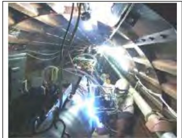
(inside of tunnel)
