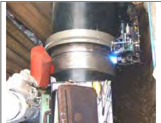
(at open cut area)
