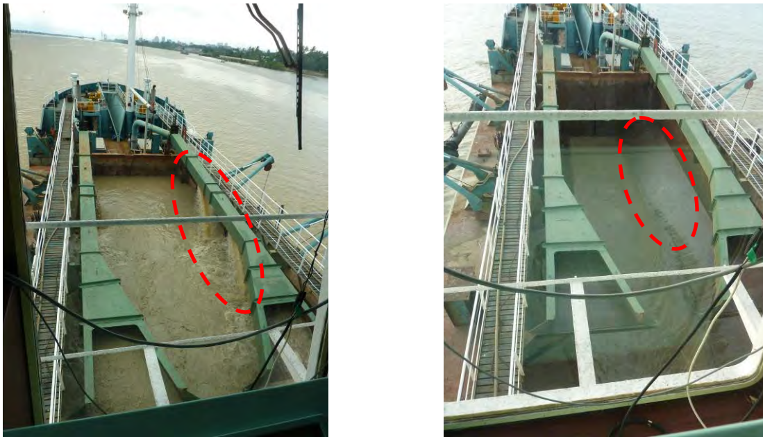
Figure 3.4-7 Dredging (Sep.28, 2012) (Pump RPM 1,100R/M)
