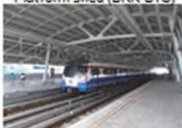
Platform shed (BKK BTS)
