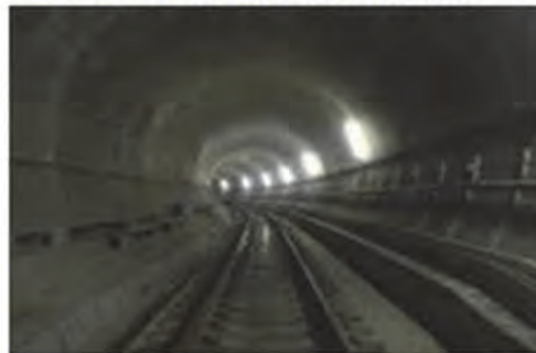
Shield Tunnel between Stations
