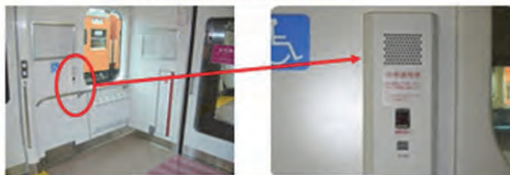
Emergency alarm device
