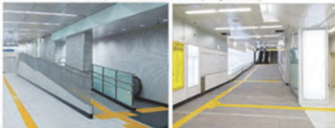
Ramp & Guidance blocks (Tokyo Metro)
