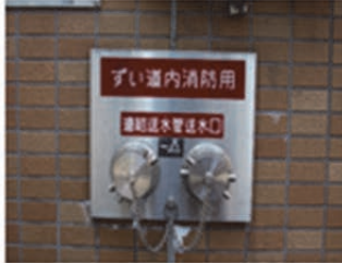
Water spray with connected water pipes
