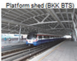
Platform shed (BKK BTS)
