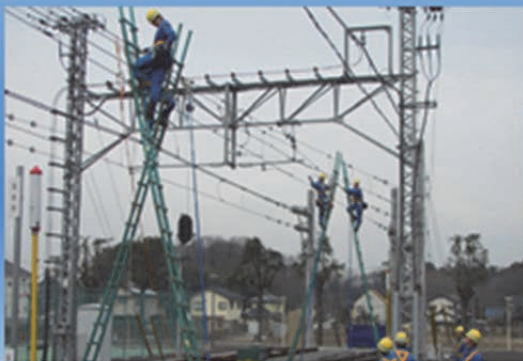
Training of contact wire recovery at the electric power maintenance depot
