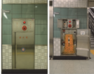
Water spray with connected water pipes
