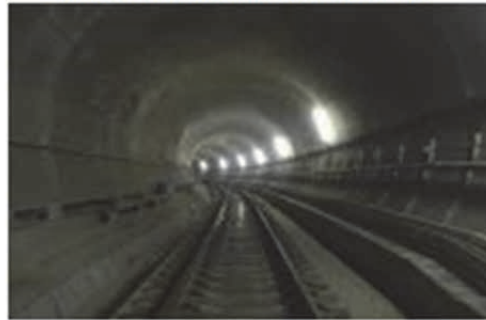
Shield Tunnel between Stations
