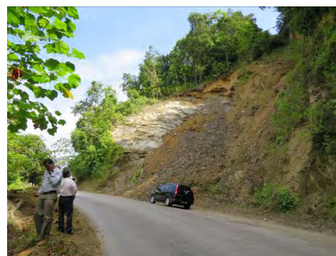
Figure 2.10.7 Slope Collapse in North Coast Road in the Trinidad Island
