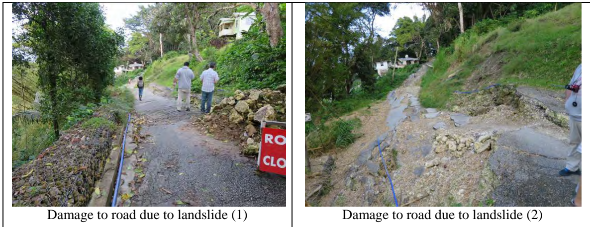
Figure 2.11.8 Damages to Roads due to Landslide in November 2014 (White Hill Area)
