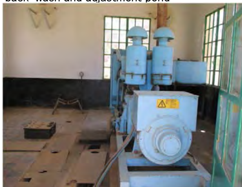
S.V W.T.P Generator is unused for the generation capacity which pump cannot work.
