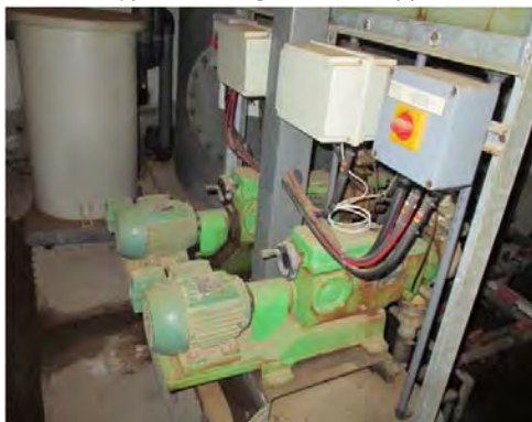
Toker W.T.P Chemical pump of chlorine liquid
