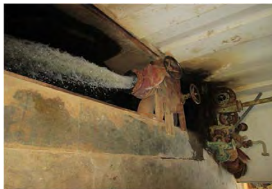
S.V W.T.P Sludge valve of back-wash
