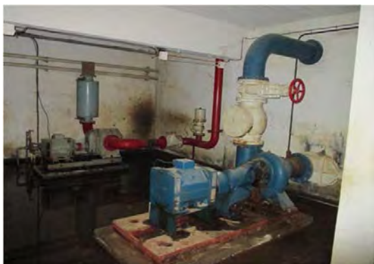
Mai Nefhi W.T.P Back-wash and air-blow pumps The opening and shutting of each valve does not function enough.
