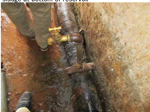
Tsetserat reservoir Water leakage from pipe
