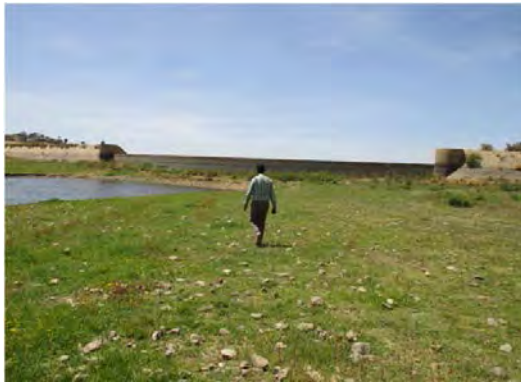
Adi Sheka dam In dam lake There is a lot of sedimentary soil in dam lake.
