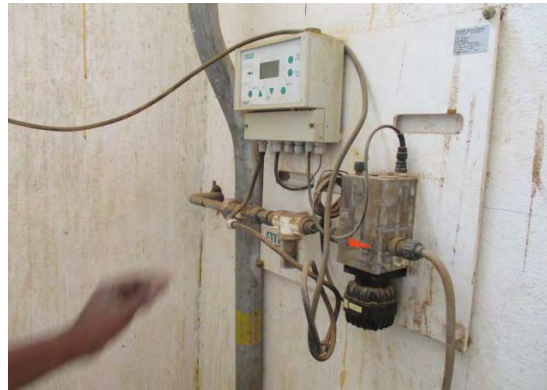
Mai Nefhi W.T.P Former chlorine gas house Old chlorine gase injector
