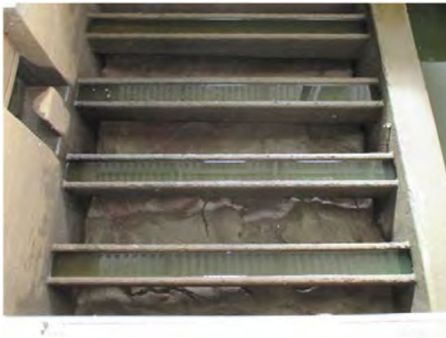
S.V W.T.P Filtration basin Mud is deposited on surface filter bed.
