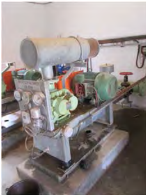
Toker W.T.P Air-blow pump
