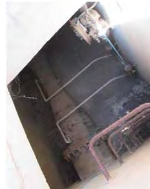
Mai Nefhi W.T.P Inlet pipe Broken Venturi equipment
