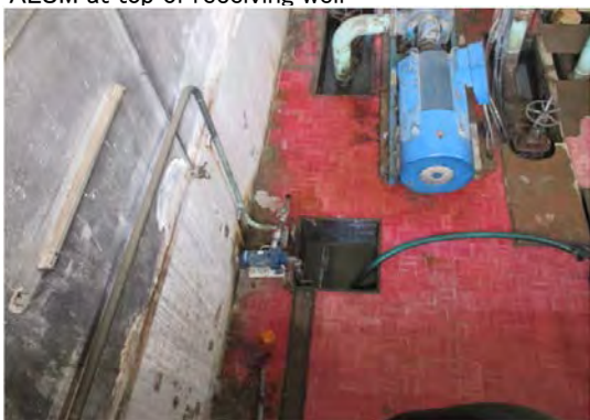
Mai Nefhi W.T.P Water leakage is discharged by a small pump.
