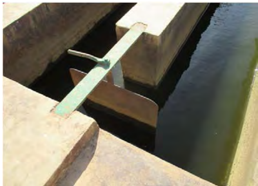
S.V W.T.P Deflector of flocculation basin It is non-operation by corrosion.
