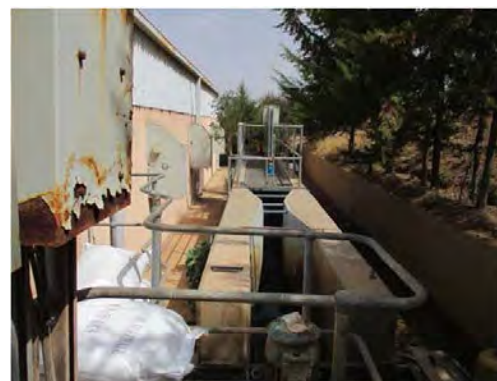
Toker W.T.P Inlet from adjustment pond Parshall flume
