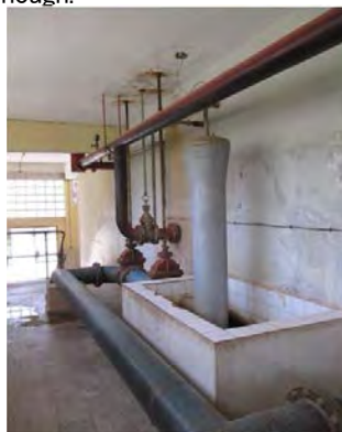
Mai Nefhi W.T.P Filtration basin of Aquazur Bottom of the basin Broken siphon The opening and shutting of each valve does not function enough.
