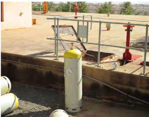
Toker W.T.P Chlorine gas Chlorine gas is injected directly into clear water reservoir.
