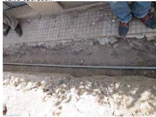
Service pipe corrugating pipe repairing
