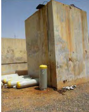
Mai Nefhi W.T.P Chlorine gas Chlorine gas is injected directly.
