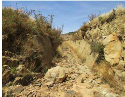
Open channel at Adi Sheka dam–Beleza dam There are a lot of falling rocks in channel.
