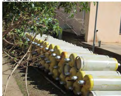
Toker W.T.P Chlorine gas cylinders piled up.
