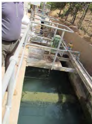
Toker W.T.P Mixing basin No.1& No.2
