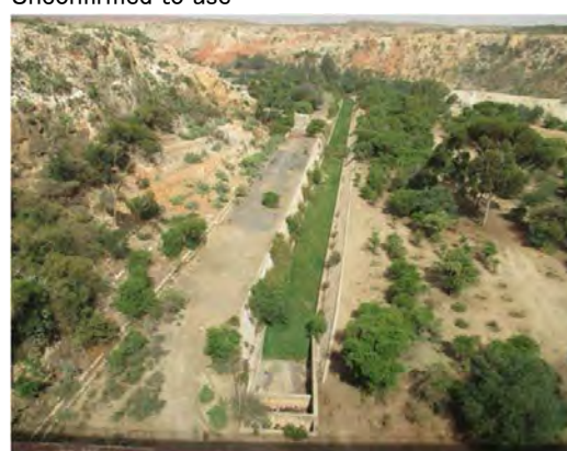
Mai Nefhi dam Channel for sludge discharge
