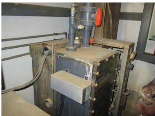
Toker W.T.P Sodium hypochlorite generation apparatus
