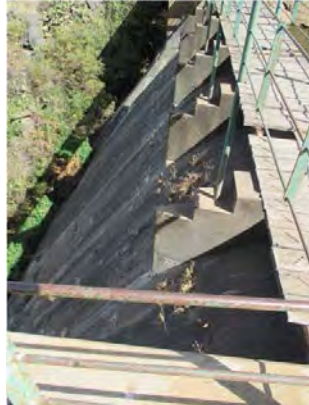
S.V dam Concrete gravity dam There seems to be enough quantity of water as of April, 2015, but there is not the water level because there is much sedimentary soil.
