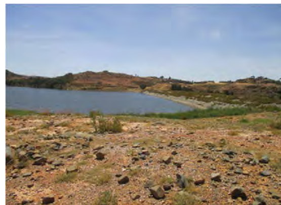
Adi Sheka dam Slope of dam of Upstream side Surface lock is protected slope of dam.
