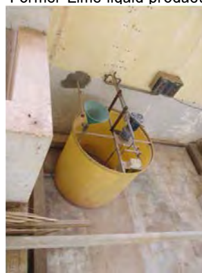
Mai Nefhi W.T.P Old chemical dosing equipment Former Polymer liquid production
