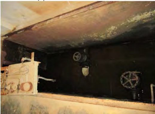
S.V W.T.P Sludge valve of back-wash etc.
