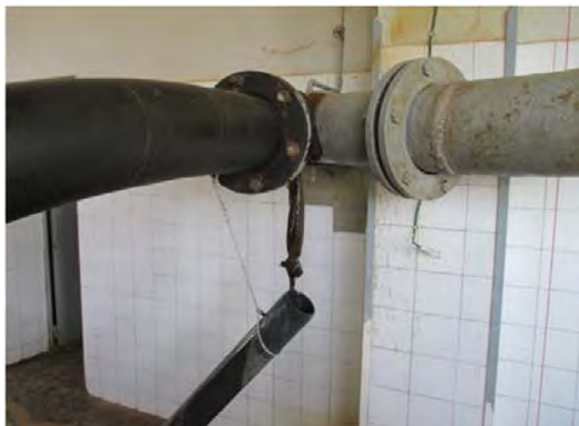
S.V W.T.P Clear water transmission pipe Water leakage from the pipeconnection
