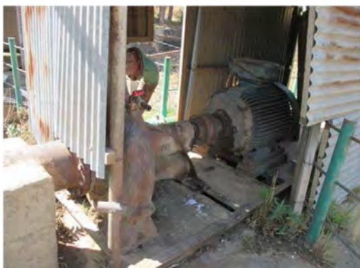
S.V dam Intake pump Intake pump on top of dam body is working.
