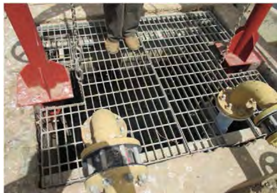
Toker W.T.P Submersible pump of wastewater pond
