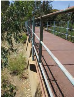
Mai Serwa dam Old spillway After downstream side collapse, spillway is unused.
