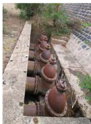
Mai Nefhi dam Valve of Sludge pipe Unconfirmed to use
