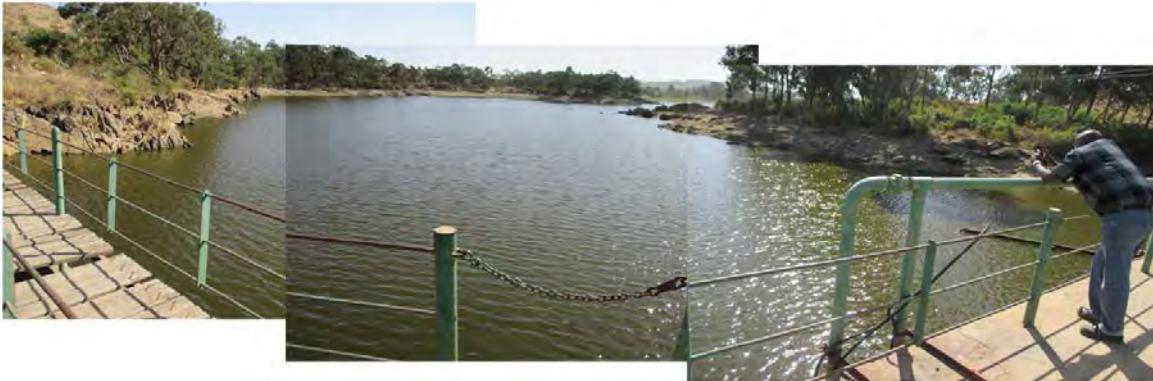
S.V dam Concrete gravity dam There seems to be enough quantity of water as of April, 2015, but there is not the water level because there is much sedimentary soil.
