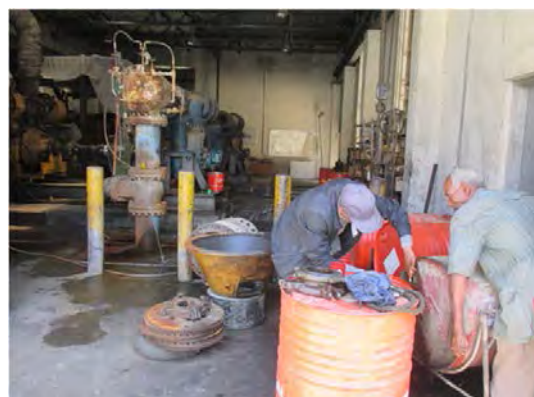
Toker raw water engine pump Oil exchange by AWS staff.
