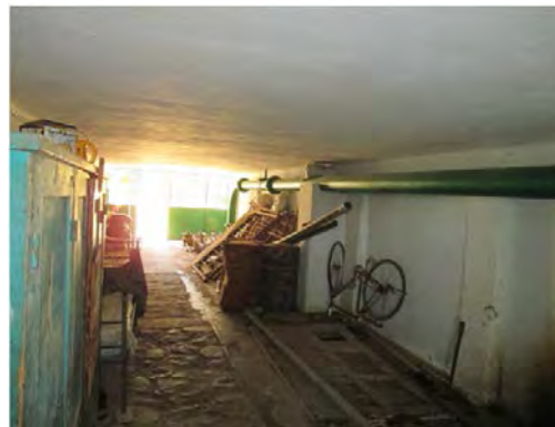
S.V W.T.P Clear water transmission pipe
