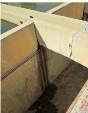
Mai Nefhi W.T.P Link channel Water leakage
