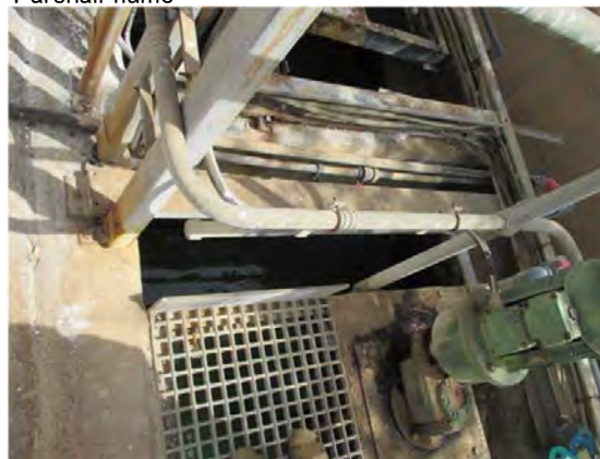
Toker W.T.P Mixing basin No.1 ALUM dosing point
