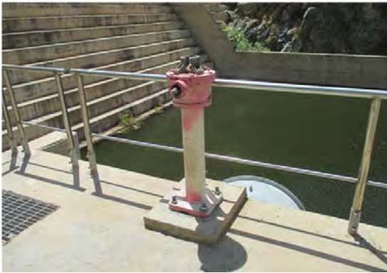
Toker dam Discharge valve
