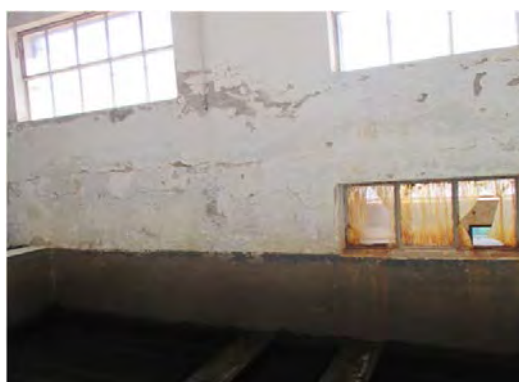
Crack and detachment of the building
