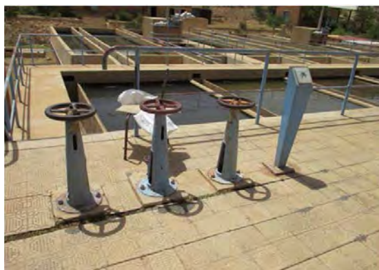
Mai Nefhi W.T.P Filtration basin of Aquazur type Broken clogging indicator
