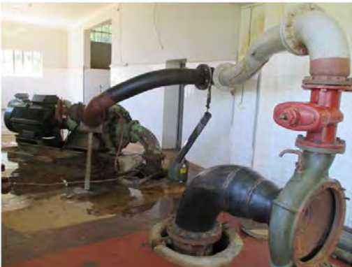
S.V W.T.P Clear water transmission pump
