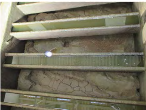
S.V W.T.P Filtration basin Hole is open on surface filter bed.
