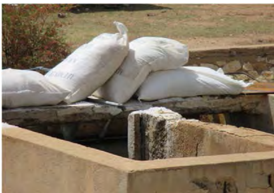
Mai Nefhi W.T.P ALUM at top of receiving well
