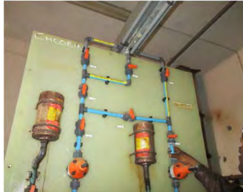
Toker W.T.P Chemical pipe of chlorine liquid
