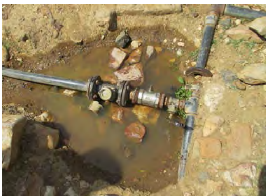
Mai Nefhi filling station Broken meter and Water leakage
