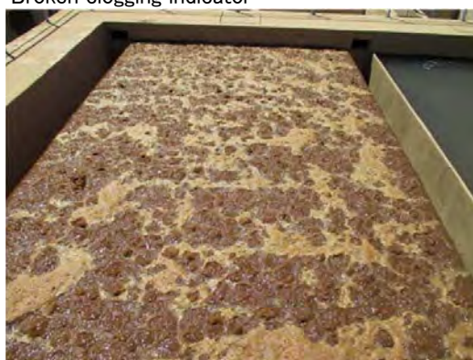
Mai Nefhi W.T.P Filtration basin of Aquazur type Backwash method, water and air at the same time are 7 minutes, water only is 8 minutes.
