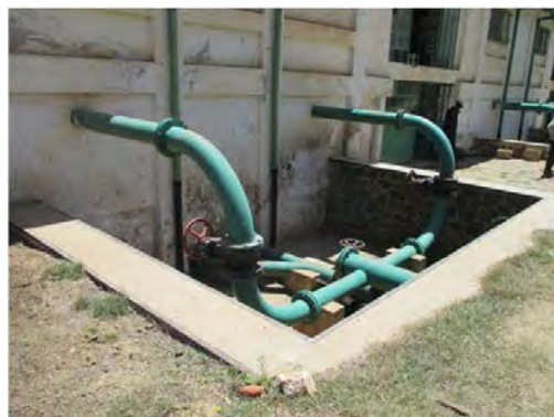
S.V W.T.P Pipe between sedimentation and adjustment pond
