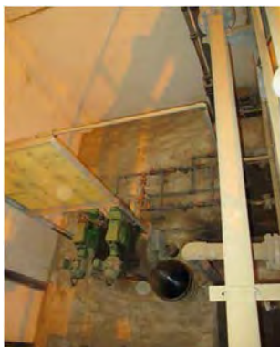
Toker W.T.P Chemical pump of ALUM
