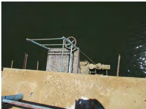
Mai Serwa dam Intake gate It has not been used in valve failure of the intake pipe.
