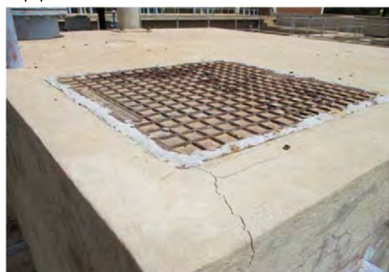
Mai Nefhi W.T.P Equipment of Vacuum tower Corroded manhole lid
