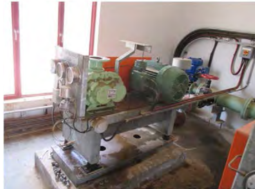
Toker W.T.P Air-blow pump
