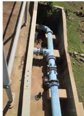
Toker W.T.P clear water transmission pipe
