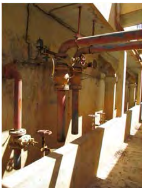
Mai Nefhi W.T.P Pulsator type flocculating sedimentation basin The opening and shutting of each valve does not function enough.
