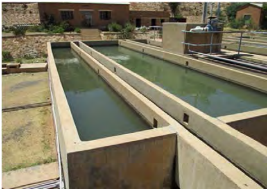
Mai Nefhi W.T.P Pulsator type flocculating sedimentation basin
