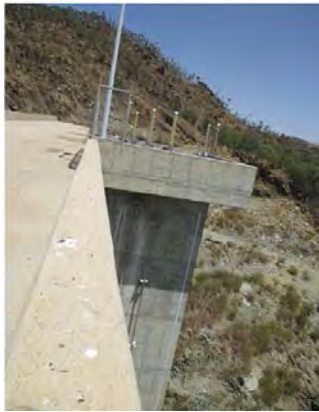
Toker dam Intake gate on dam body
