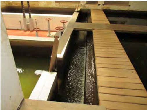
S.V W.T.P Outlet of adjustment pond
