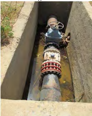
Mai Nefhi W.T.P Clear water transmission pipe Broken meter
