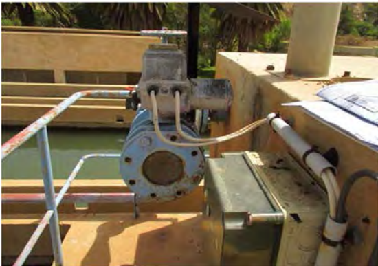
Mai Nefhi W.T.P Equipment of Vacuum tower Broken Vacuum release valve
