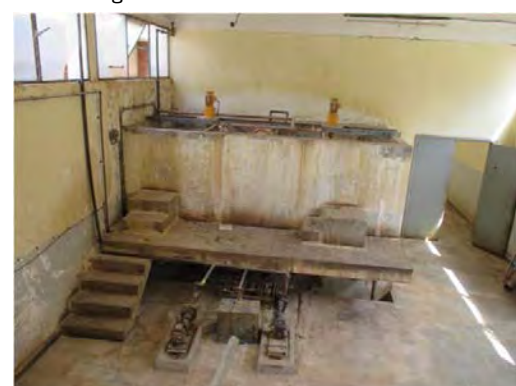
Mai Nefhi W.T.P Old chemical dosing equipment Former ALUM liquid production
