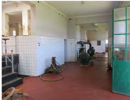
S.V W.T.P Clear water transmission pump
