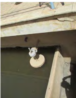
Mai Nefhi W.T.P Filtration basin of Aquazur type Broken partialization box
