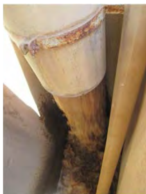
Mai Nefhi W.T.P Filtration basin of Aquazur type State of sludge water at the time of back-wash
