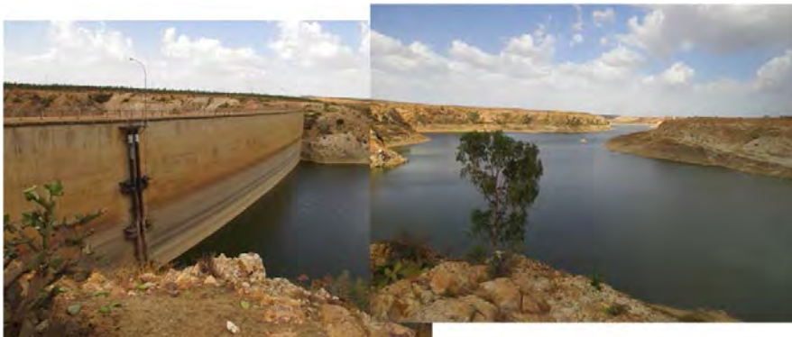
Mai Nefhi dam Concrete gravity dam
