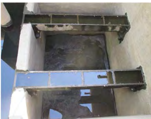
Toker W.T.P Filtration basin State of filter bed.
