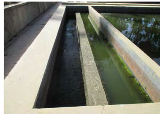
S.V W.T.P Link channel between flocculation and sedimentation basins.
