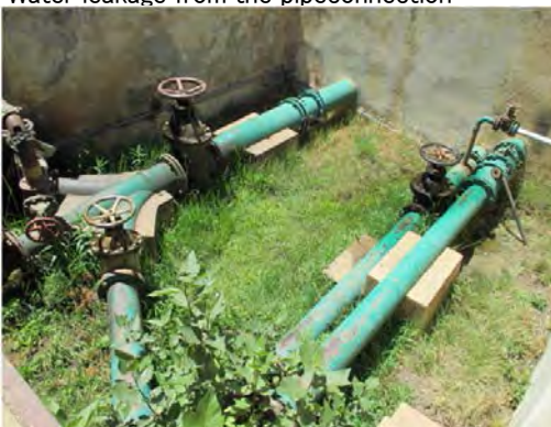
S.V W.T.P Clear water transmission pipe and back-wash pipe
