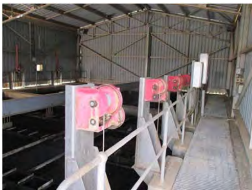
Toker W.T.P Sedimentation (Inclined plate) basin
