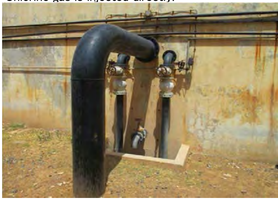
Mai Nefhi W.T.P Inlet pipe from receiving well to pulsator type flocculating sedimentation basin
