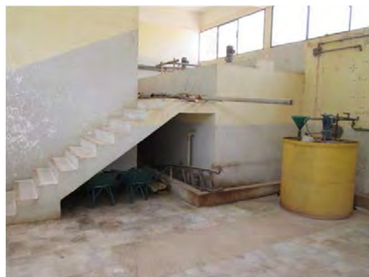
Mai Nefhi W.T.P Old chemical dosing equipment Former Lime liquid production
