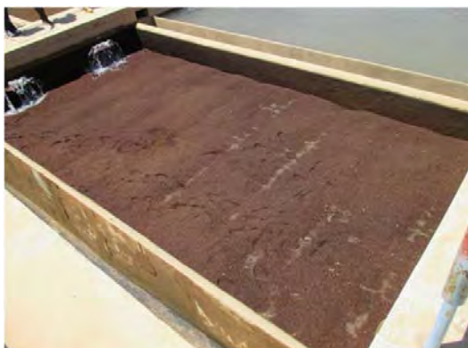
Mai Nefhi W.T.P Filtration basin of Aquazur type State of filter bed after back-wash
