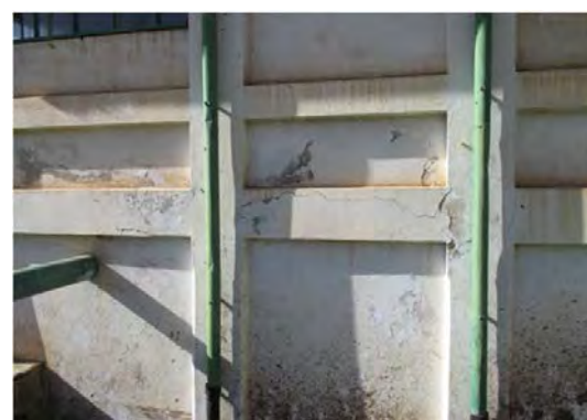
Crack and detachment of the building
