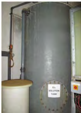
Toker W.T.P Chlorine liquid tank from Sodium hypochlorite generation apparatus
