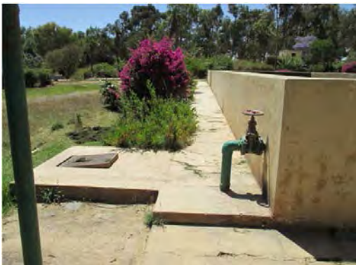
S.V W.T.P Sludge pipe of sedimentation Sludge discharge valves are out of order
