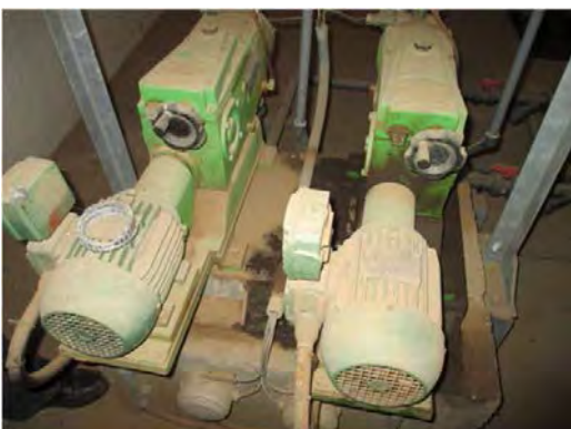
Toker W.T.P Chemical pump of ALUM
