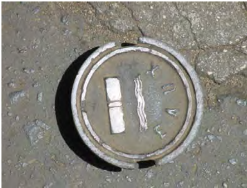
Distribution network Valve box
