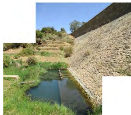
Mai Serwa dam Downstream side of dam Four valves are unusable for mud clogging among five valves of sludge pipe.
