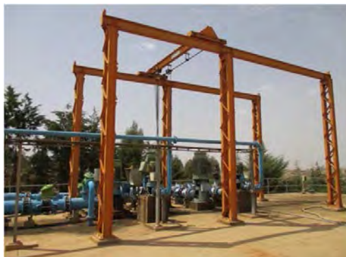
Toker W.T.P Top of Clear water reservoir Transmission pump and Back-wash pump
