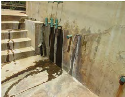
S.V W.T.P Water leakage water leakage at receiving well
