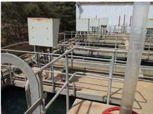
Toker W.T.P Flocculation basin
