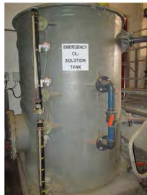
Toker W.T.P Chlorine liquid tank from hypochlorous acid powder
