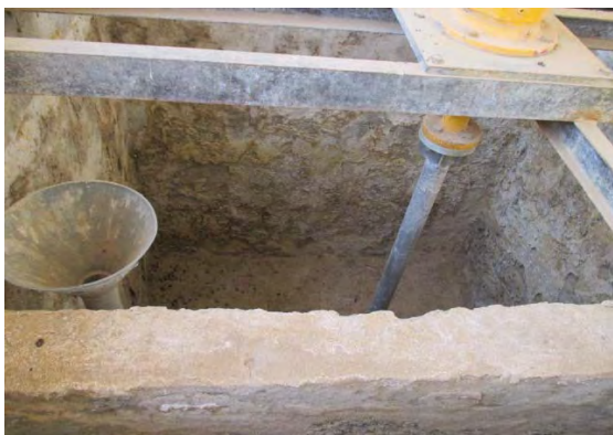
Mai Nefhi W.T.P Old chemical dosing equipment Former ALUM liquid production
