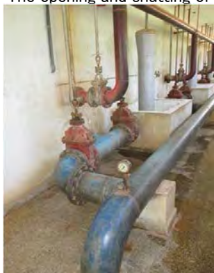
Mai Nefhi W.T.P Filtration basin of Aquazur Bottom of the basin Broken siphon The opening and shutting of each valve does not function enough.
