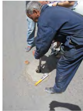
Distribution network valve operation
