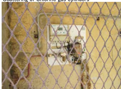
New Sembel pumping station Broken chlorine gas injector
