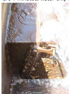
Mai Nefhi W.T.P Filtration basin of Aquazur type Broken Crack valve
