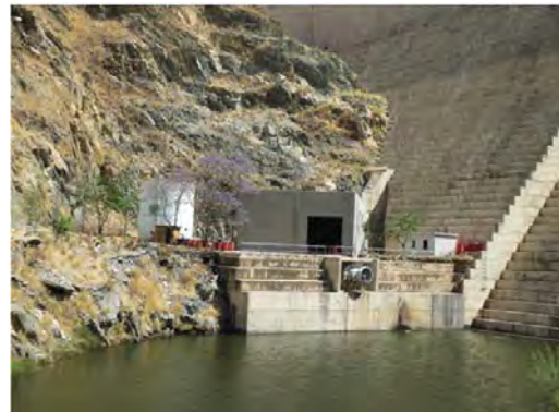
Toker dam Pump station and Discharge pipe
