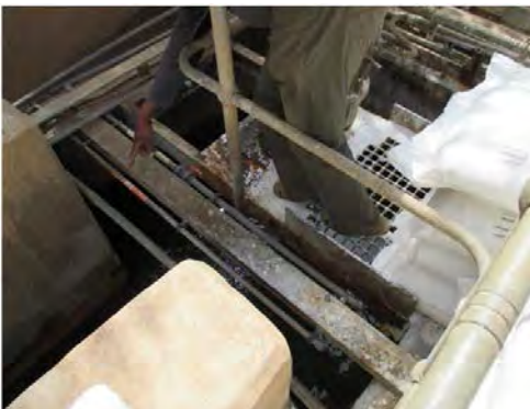
Toker W.T.P ALUM is put in directly at the time of blackout
