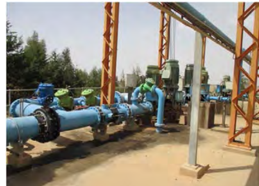
Toker W.T.P Top of Clear water reservoir Transmission pump and Back-wash pump
