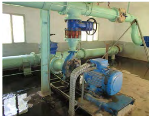
Adi Sheka raw water pump It's leaking, but it isn't repaired.
