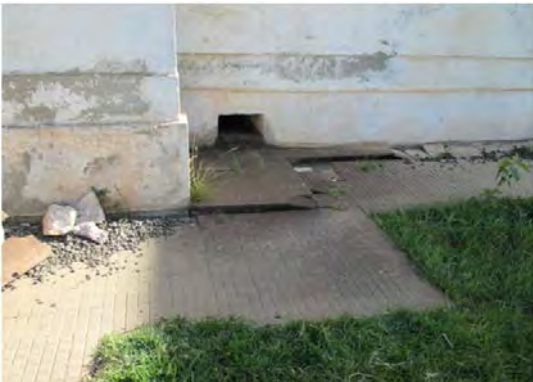
S.V W.T.P Structure of filtration basin and clear water reservoir Subsidence about 5 cm.
