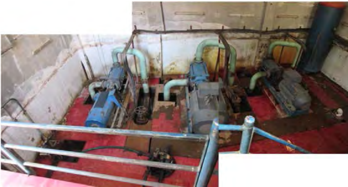
Mai Nefhi W.T.P Clear water transmission pump Water leakage
