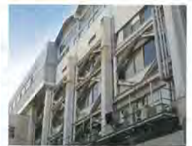
Seismic strengthening of the Hamamatsuchō Station building
