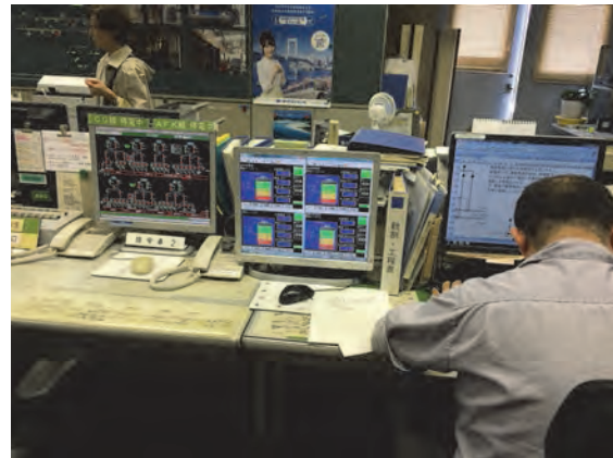
Operation Control Center 2
