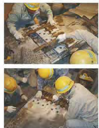
Maintenance and repair of extendable-joint striker plates
