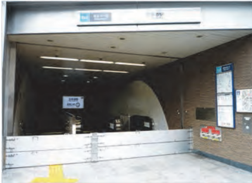
Figure 11.2.1.2-1 Removable Water-stop Panels at Station Entrance
