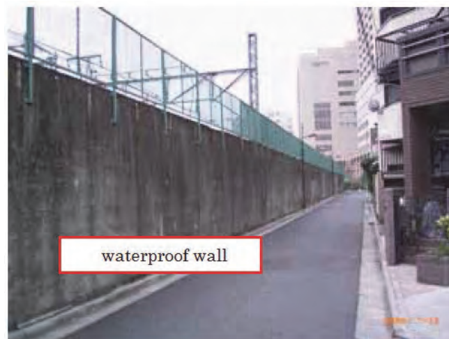
Figure 11.2.1.2-6 Waterproof Wall at Grade Section (outside measure)
