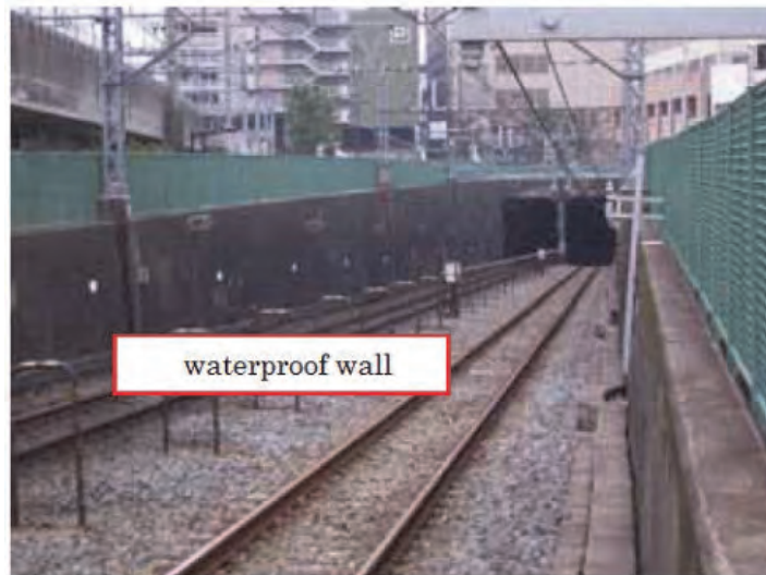
Figure 11.2.1.2-7 Waterproof Wall at Grade Section (inside measure)
