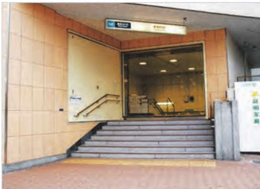
Figure 11.2.1.2-2 Flood Prevention Iron Door at Raised Station Entrance
