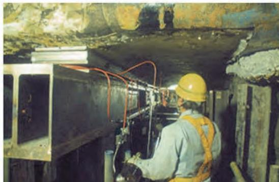
Flat jack inserted between building frame and beam
