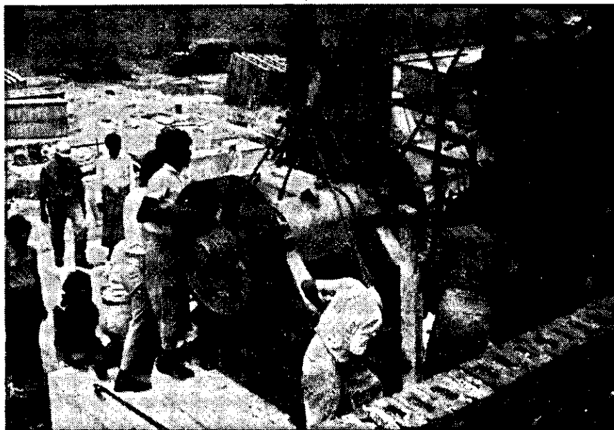
CRUSHER SETTING AT MILL-SITE BY A CRAWLER-CRANE
