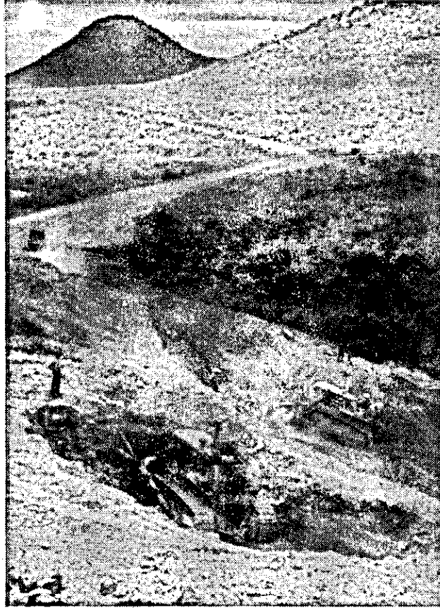
OVERBURDEN STRIPPING BY BULLDOZERS JUNE 6, 1975
