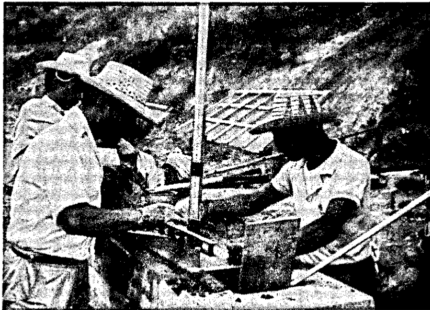
CAREFUL SETTING OF THE BASE PLATE FOR A BALL MILL
