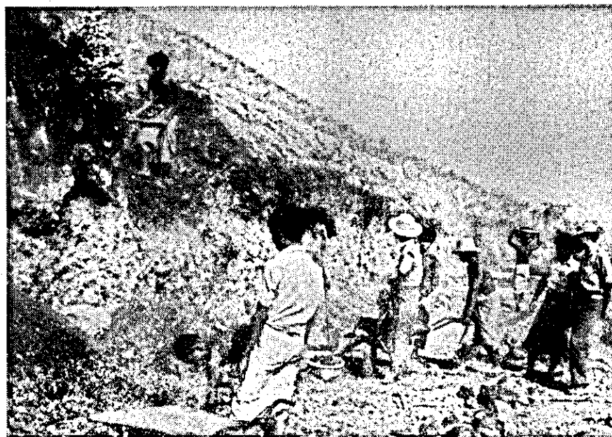
PRELIMINARY WORK STARTED IN APRIL, 1975 "MILL SITE CONSTRUCTION"
