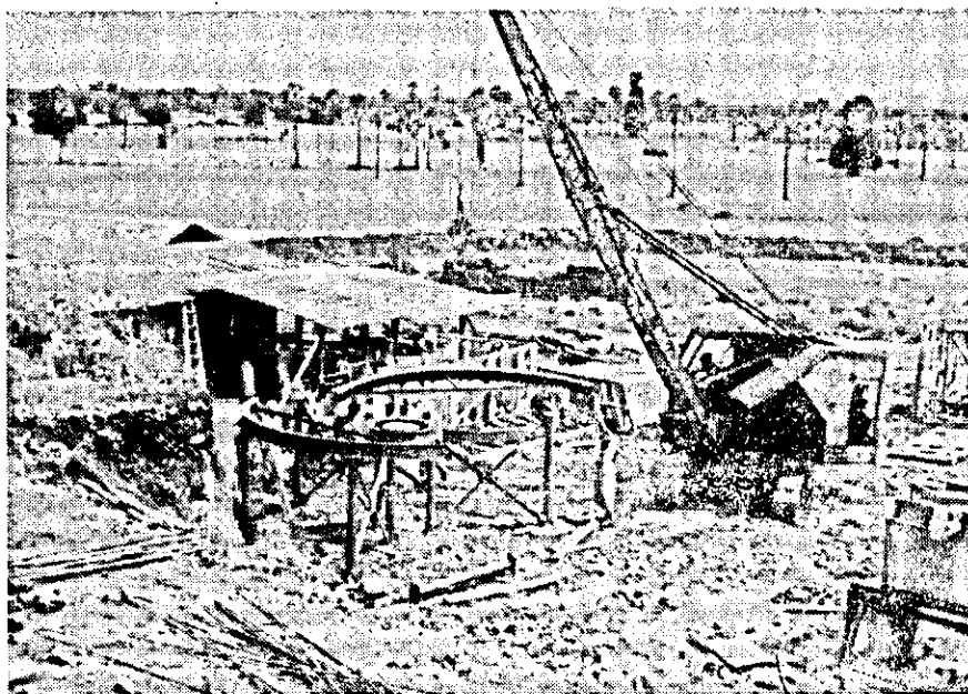
SETTING OF BASAL FRAME OF A THICKENER "TAILING POND IN BACKGROUND"
