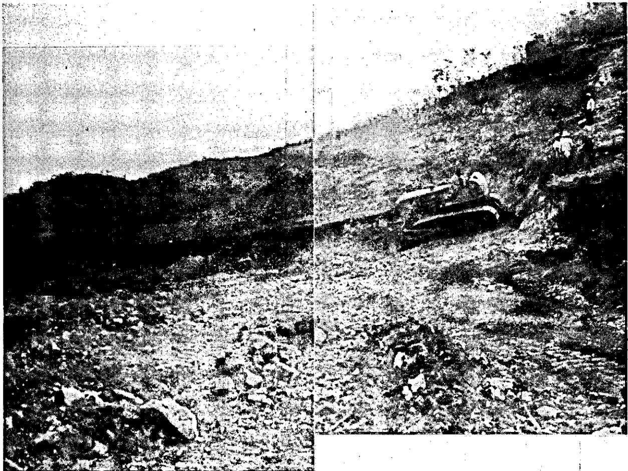
CLEARING OF STRIPPING SITE SABEDAUNG JUNE, 1975
