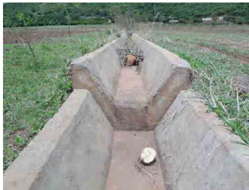
Canals constructed by DOI in Block A
