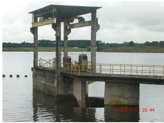
4. Intake of Piraquara Dam II
