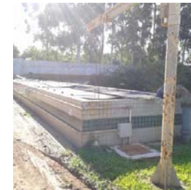
Image 11 - Final Effluent Outfall
