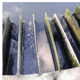
Image 33 – Diffuser beak obstructed
