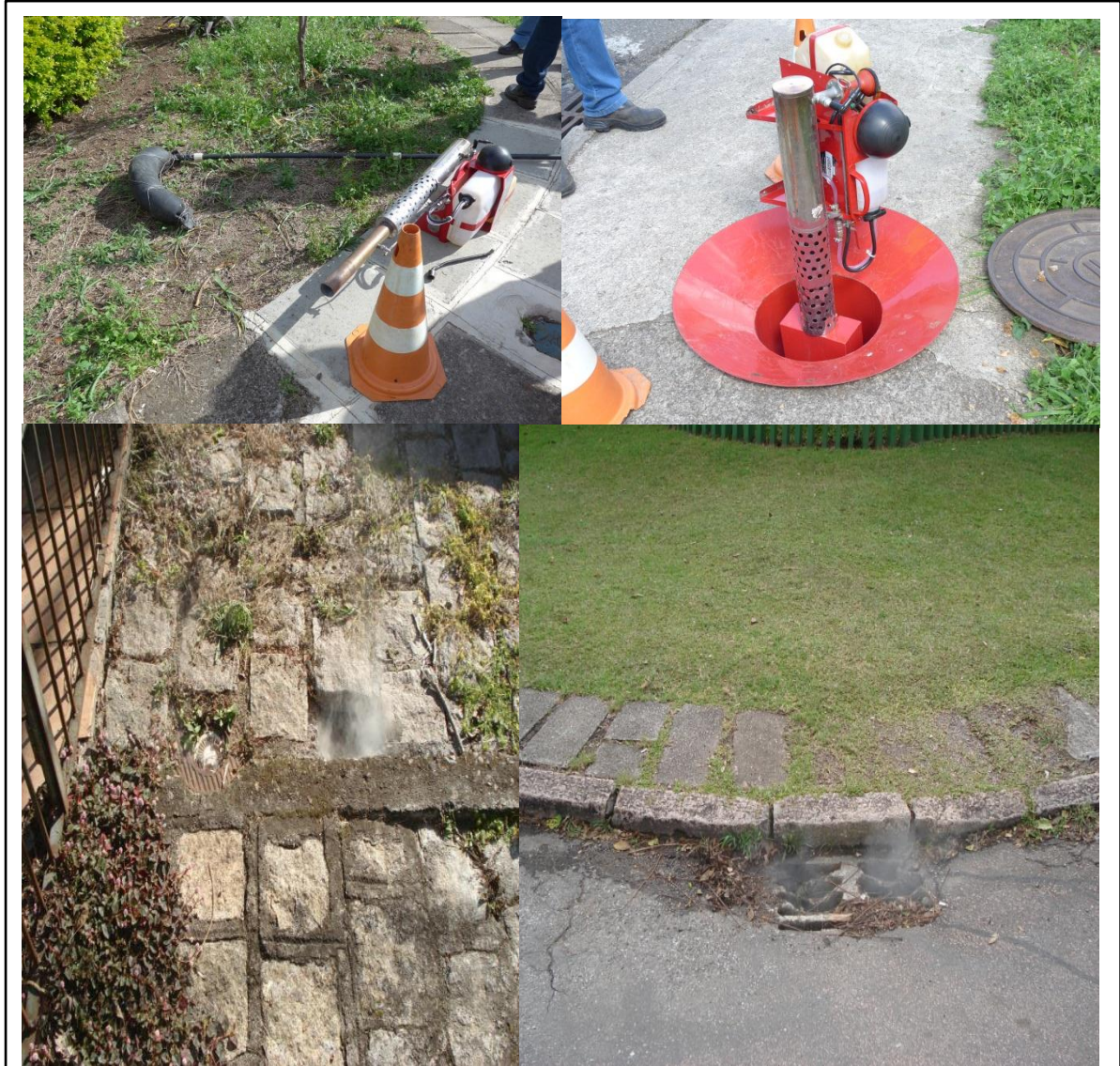
Photograph 4-1 Implementation of Smoke Test
