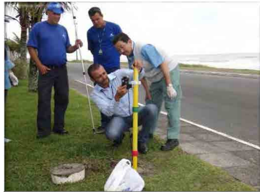
OJT for Site Investigation with TV Camera
