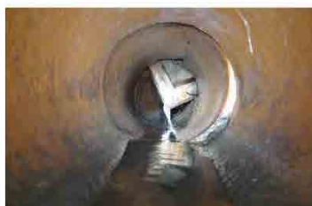
Injection of house connection
