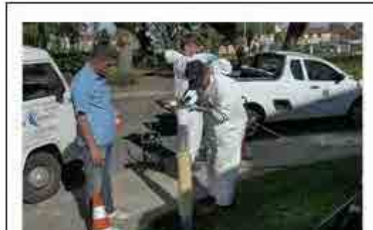
Demonstration construction of pipe rehabilitation method
