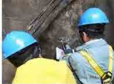
Drilling side wall
