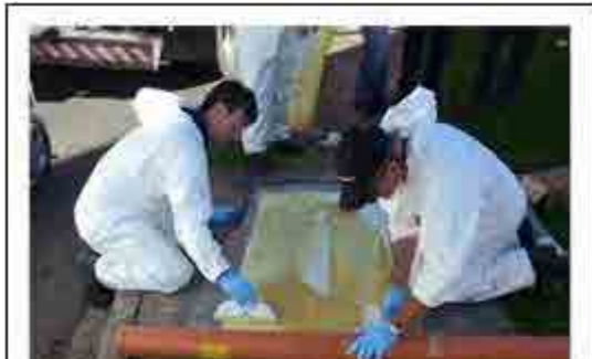
Demonstration construction of pipe rehabilitation method
