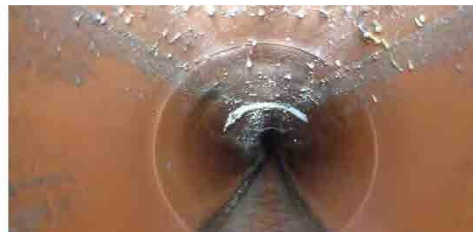
Sewage pipe without problem
