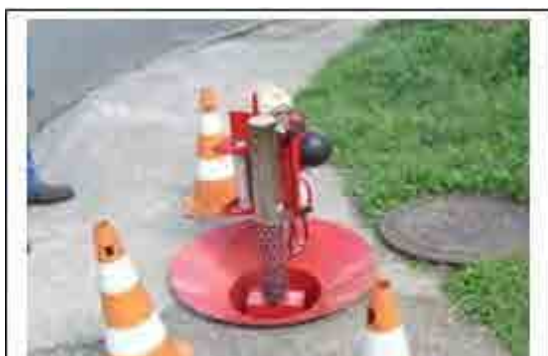
Equipment for smoke test
