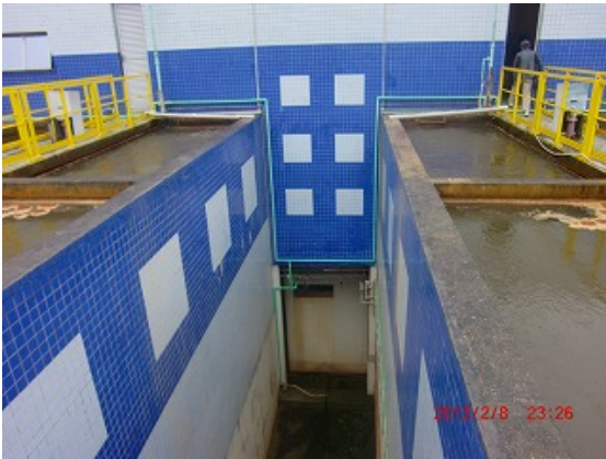
7. Flocculator of Irai WTP (Coagulant: \text{Al}_2(\text{SO}_4)_3 )
