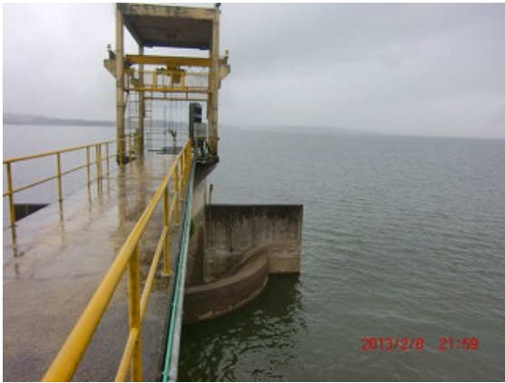
3. Intake of Irai Dam
