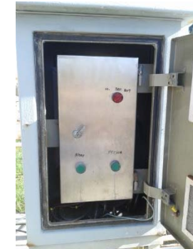
Image 56 - Bypass sluice panel
