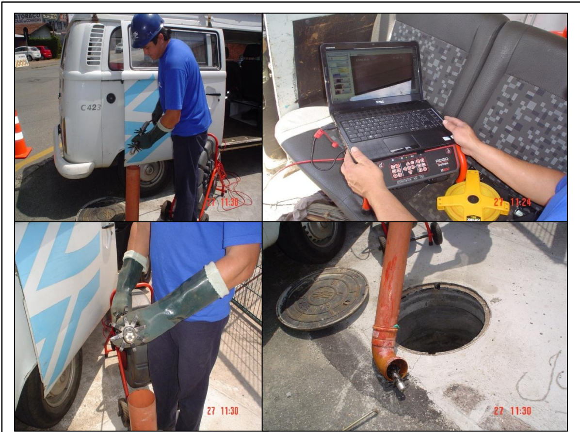
Photograph 3-2 Field Investigation by Insert-Type TV Camera
