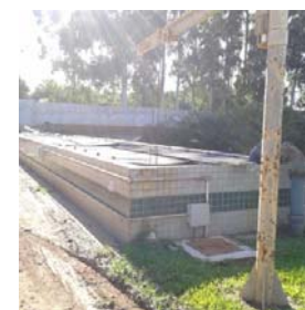
Image 11 - Final Effluent Outfall
