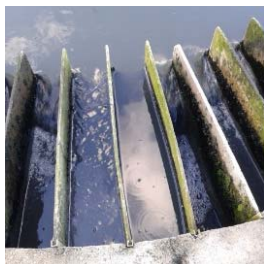
Image 33 – Diffuser beak obstructed
