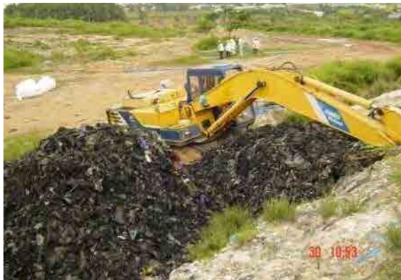
a. Crane used for excavating and taking SW in landfill cell
