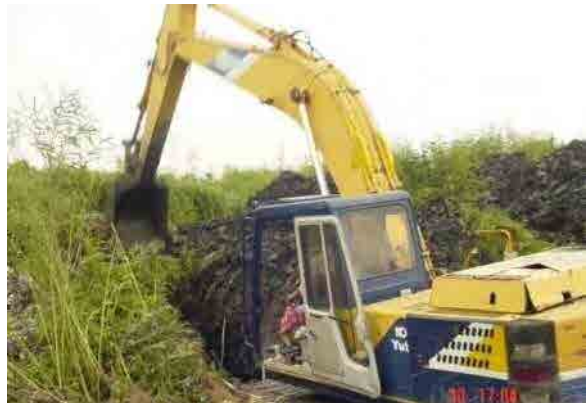
a. Crane used for excavating and taking SW in landfill cell
